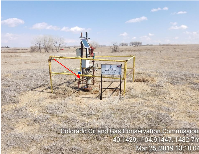
Photo 1 WH. Appears to be a leak on 1/4 gas line to drip pot
