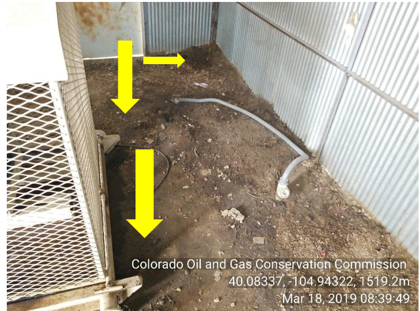
Photo 18 Stained soil inside pump house
