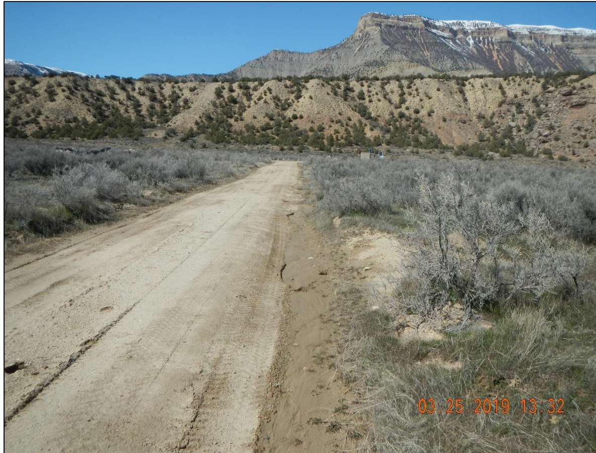
Sediment build up in ditches.
