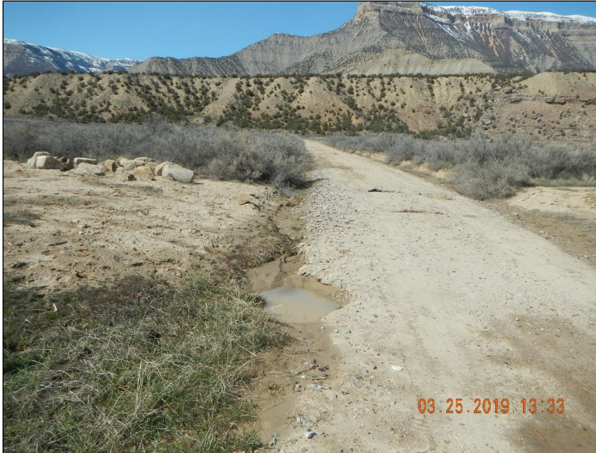
Sediment build up in ditch.
