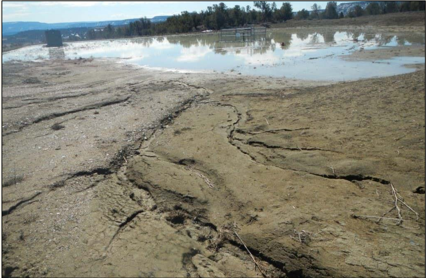
Photo 1. View of the project area from the project entrance facing center. Erosion is occurring at the entrance and water is ponded on the well pad.
