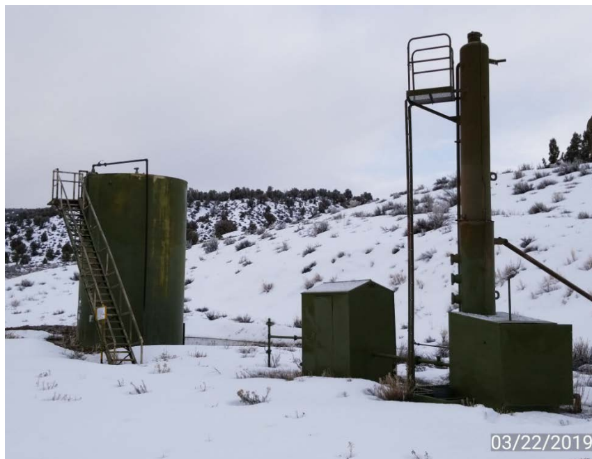
Photo 5. Crude tank, gas building, vertical separator.
