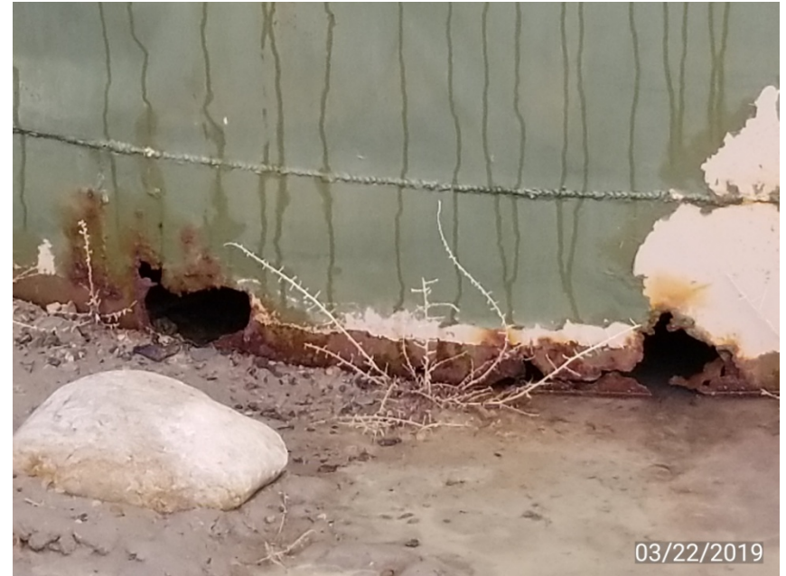
Photo 4. Water tank with holes at base.
