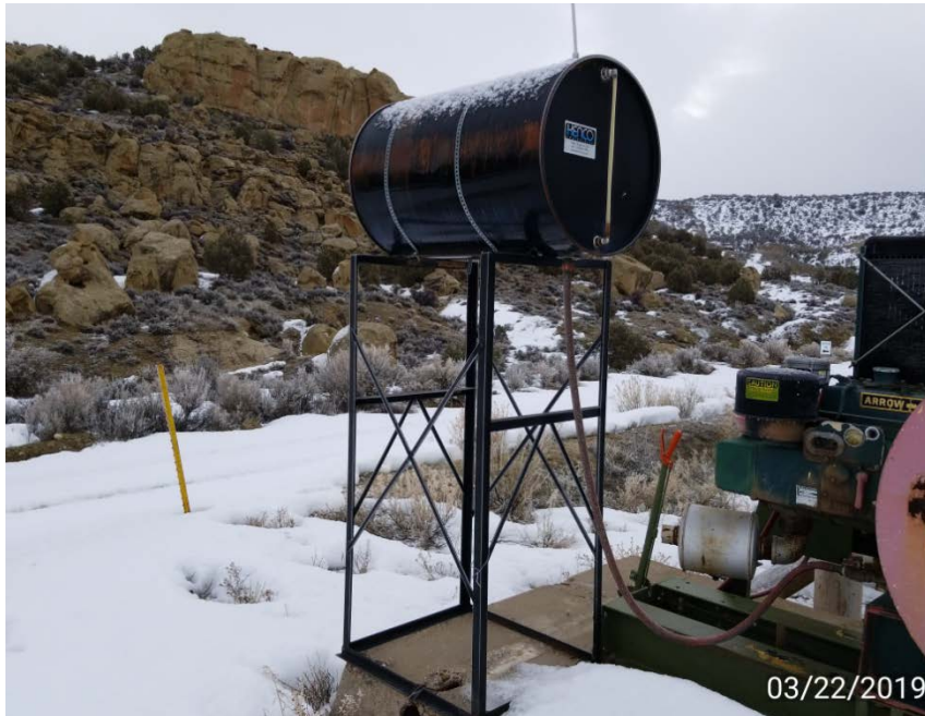
Photo 7. Container without contents label & secondary containment.
