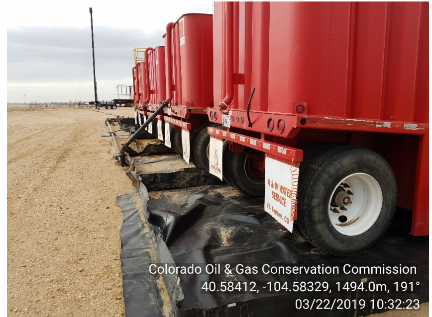
Photo #2 Temporary flowback tanks. Corrective Action: Flowback tanks do not appear to be grounded.
