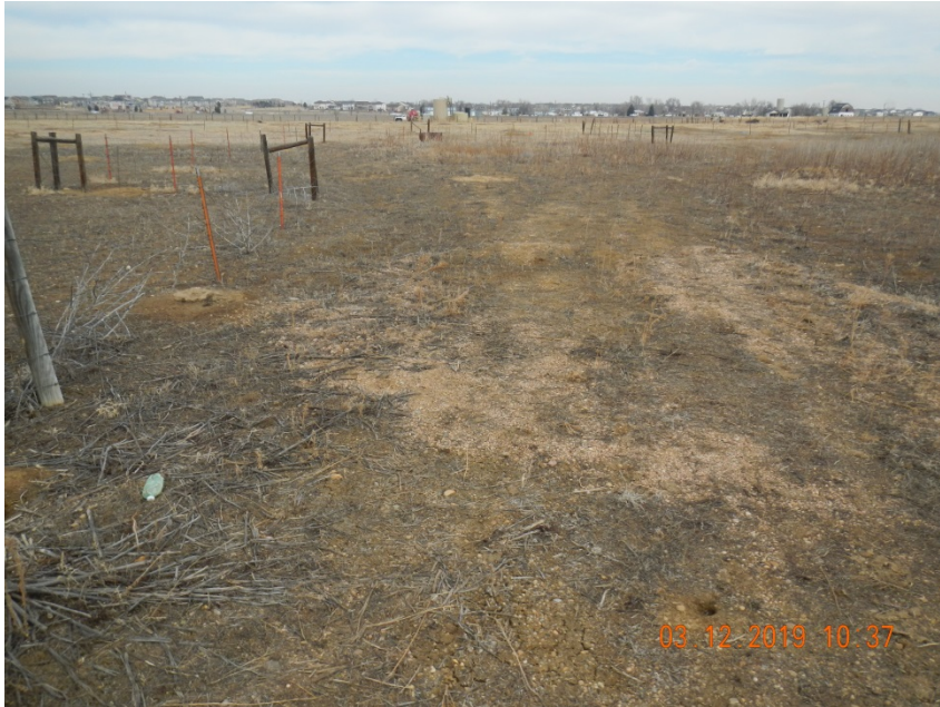
Photo 1. Photo taken from the access road off, facing North. Photo depicts the access road remains on location, the gravel has not been removed and has not been re-contoured or re-graded and decompacted to meet the adjacent terrain.
