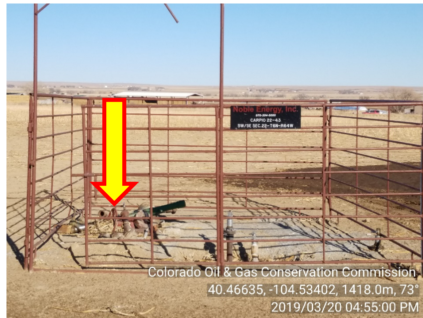
Photo #2 Carpio 22-43 Wellsite Plugged & Abandoned | PA Wellhead NOT cut & capped Unused Equipment
