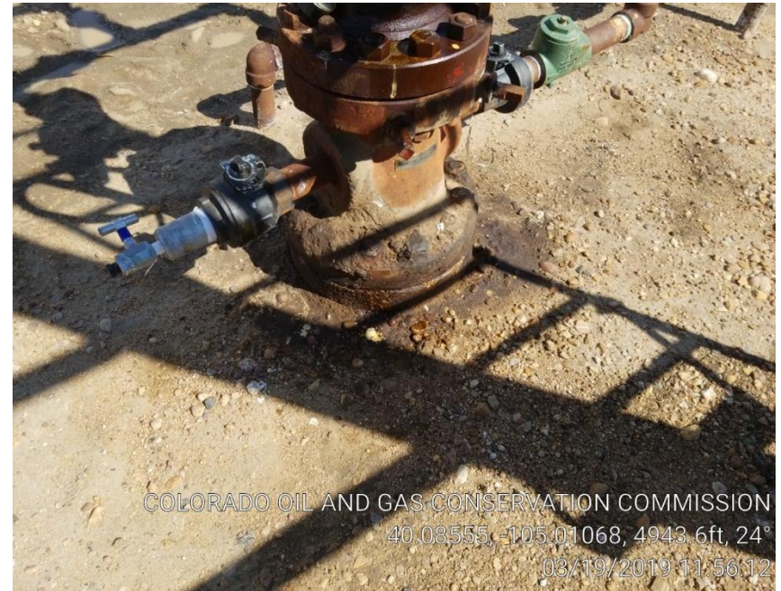
Pic 4 possible leak
