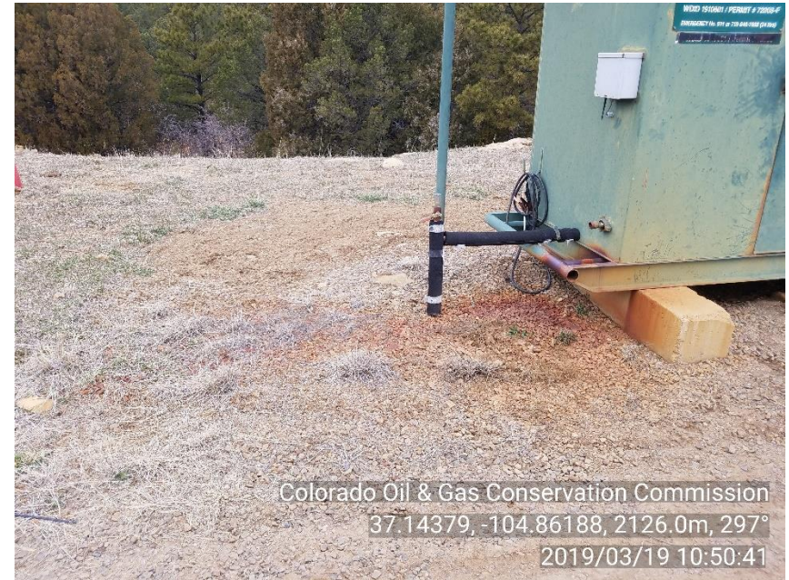
PHOTO 4: IMPACTED SOIL NEAR SEPARATOR DRAIN ON METER HOUSE
