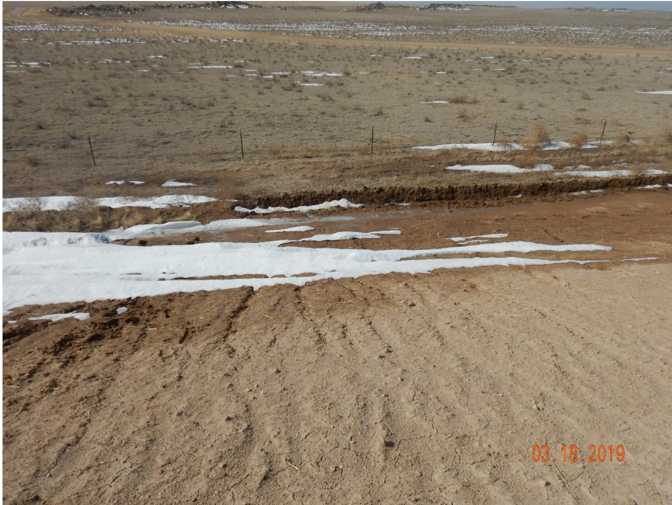
Photo 2: Photo taken from the south end of the pad, facing south. Photo shows section of stormwater ditch where discharge was occurring has been repaired to mitigate runoff.
