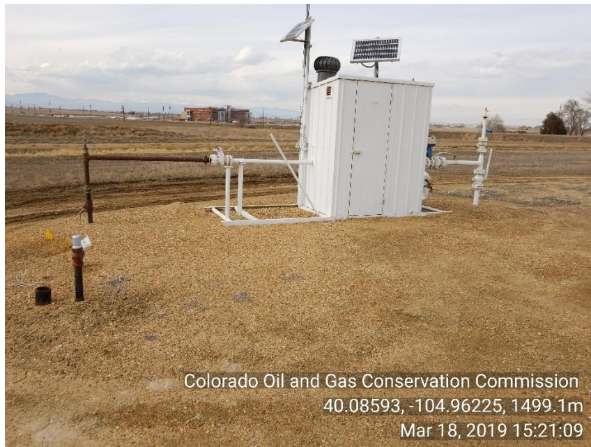
Photo 3 Meter house. Riser is bull plugged and marked
