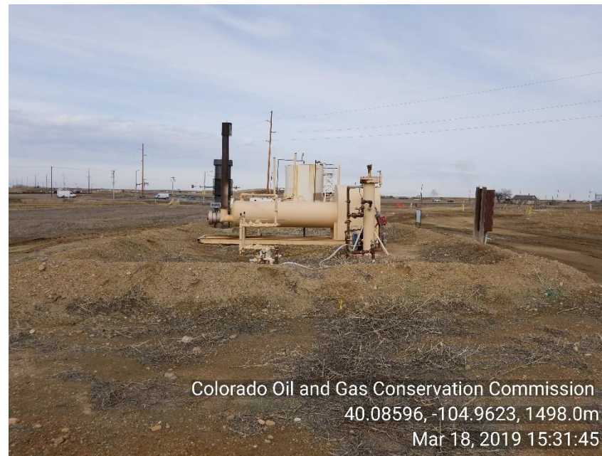
Photo 6 ECD, separator and compressor
