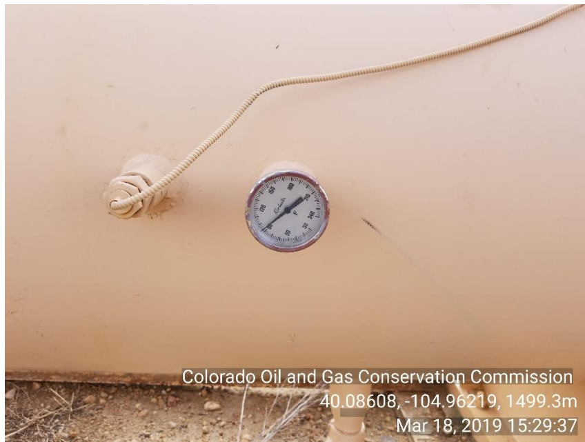
Photo 5 Separator appears to have approximately 90psi
