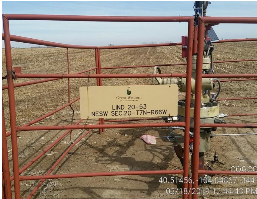
Photo – 1 Wellhead Sign missing Emergency Contact Info
