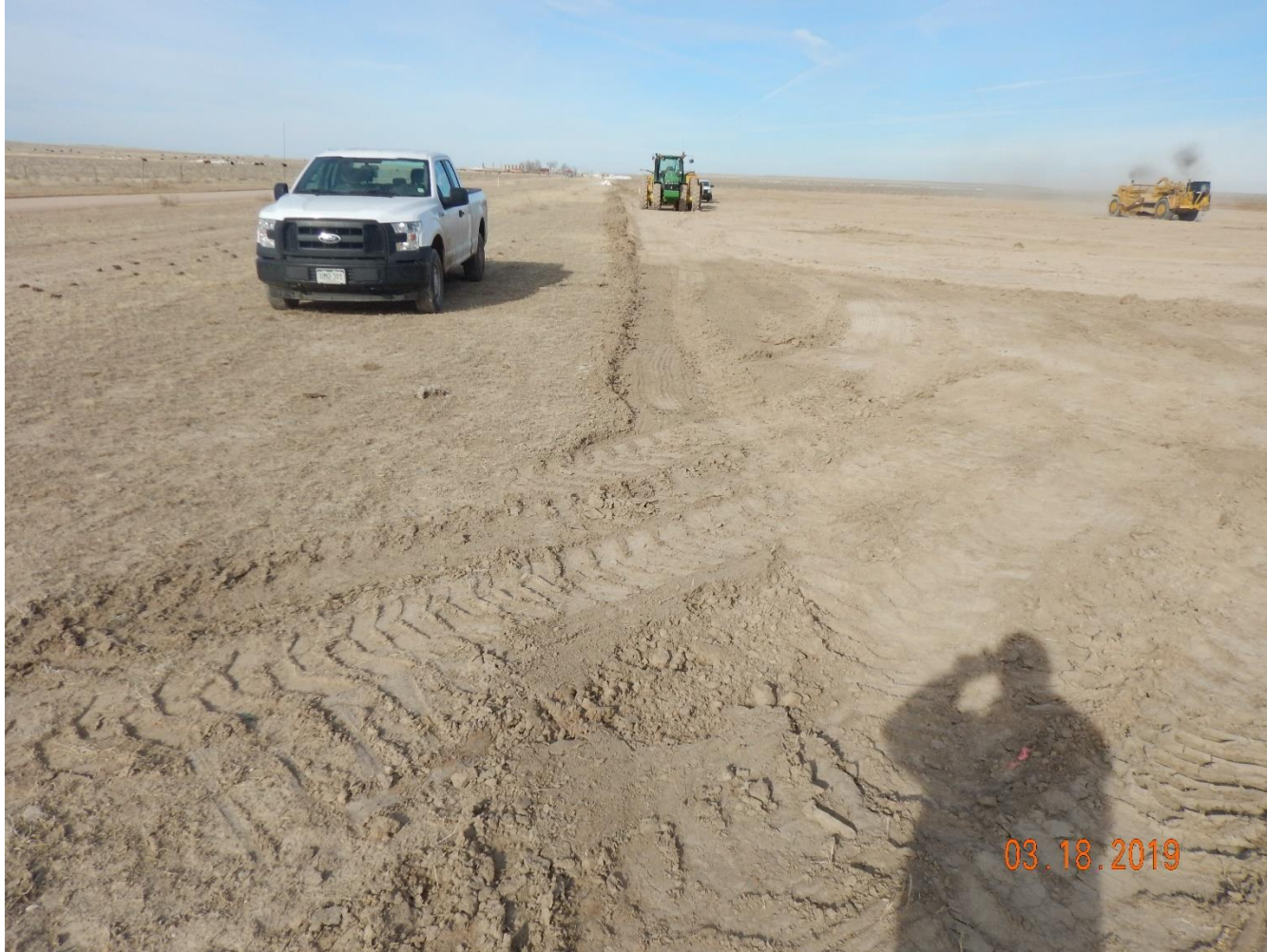
Photo 1: Photo taken from the southeast corner of the location, facing west. Photo provides overview of construction in-process. Photo also shows operator failed to install perimeter stormwater and erosion control BMPs prior to construction activities in accordance with Rule 1002.f and COAs from the permitted 2A
