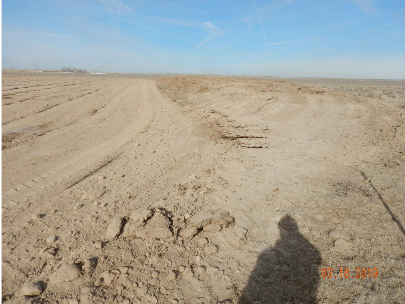
Photo 3: Photo taken from the northeast end of the location, facing west. Photo shows topsoil stockpile. Ensure BMPs are implemented to protect stockpiled soils in accordance with 1002.c
