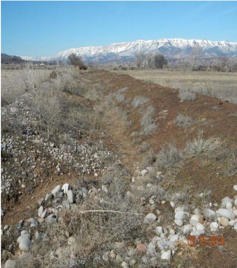
Photo#8: Berm needs to be stabilized.
