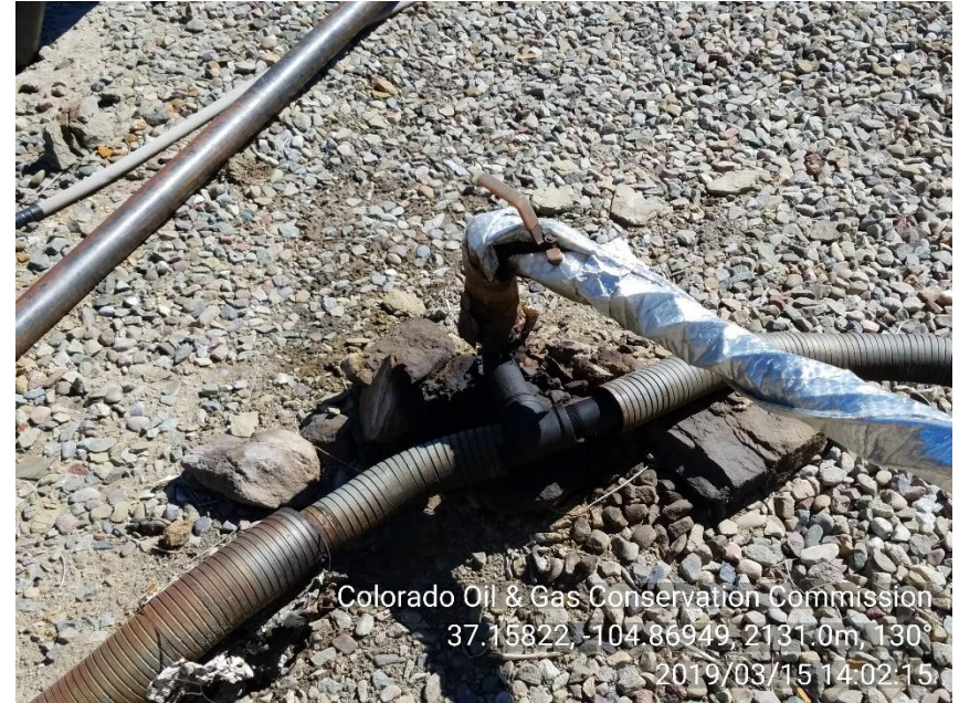
PHOTO 4: IMPACTED SOIL NEAR EXHAUST PIPE ON EAST SIDE OF ENGINE SKID.
