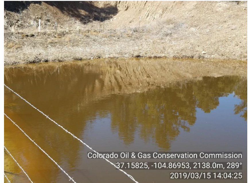
PHOTO 6: ANOTHER VIEW OF PRODUCED WATER LEVEL ABOVE 2' FREEBOARD.
