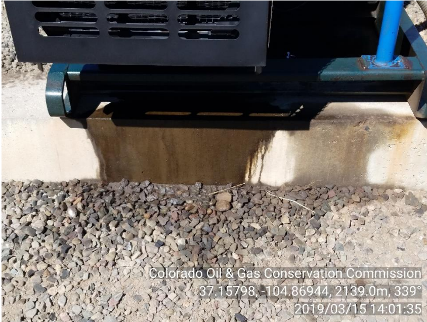
PHOTO 3: OIL FROM ENGINE IS RUNNING DOWN CONCRETE BLOCK AND IMPACTING SOIL.
