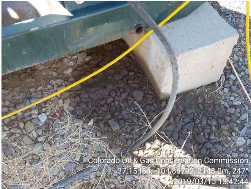
PHOTO 3: IMPACTED SOIL ON EAST SIDE OF ENGINE SKID
