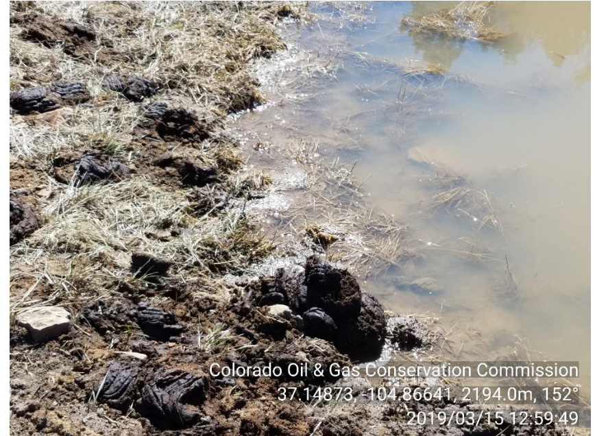
PHOTO 3: PRODUCED WATER IN PIT IS ABOVE THE 2' FREEBOARD.
