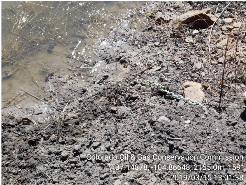
PHOTO 7: FREEBOARD MARKER IS IMPROPERLY INSTALLED ON THE HIGHER ELIVATION SIDE OF PIT.
