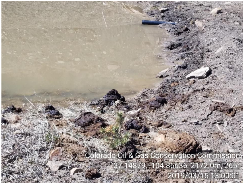
PHOTO 5: PRODUCED WATER IN PIT IS ABOVE THE 2' FREEBOARD.
