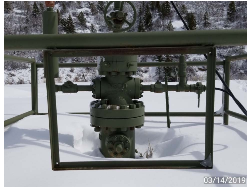
Photo 2. No wellhead sign.
