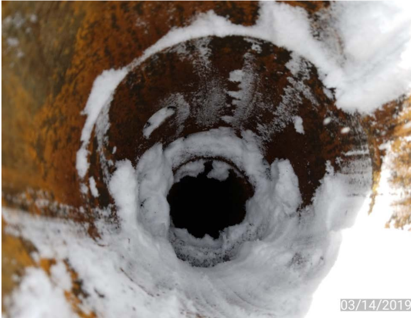
Photo 3. Looking down into wellhead casing.
