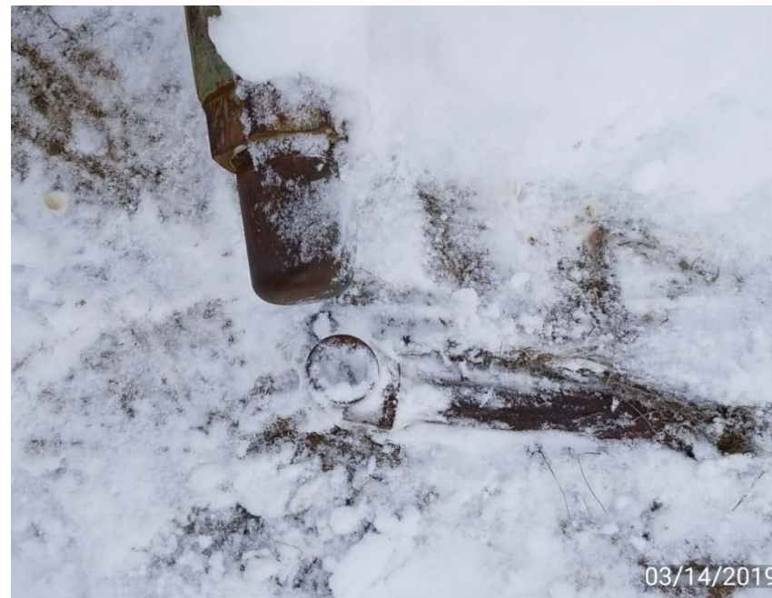
Photo 2. Uncapped riser next to wellhead.
