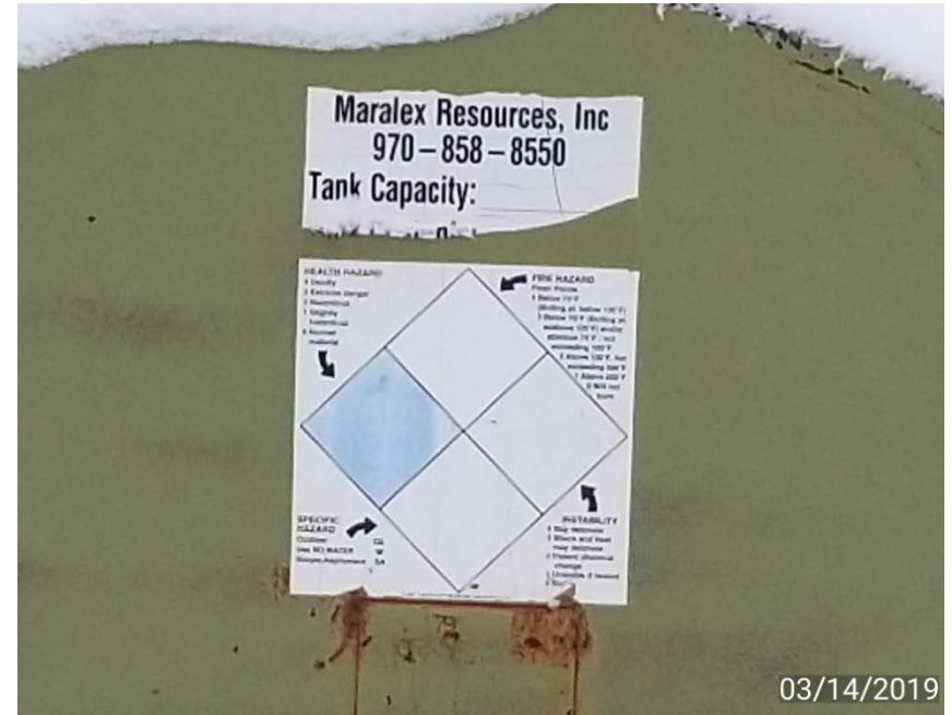
Photo 2. Tank label with blank capacity, contents, and NFPA label.
