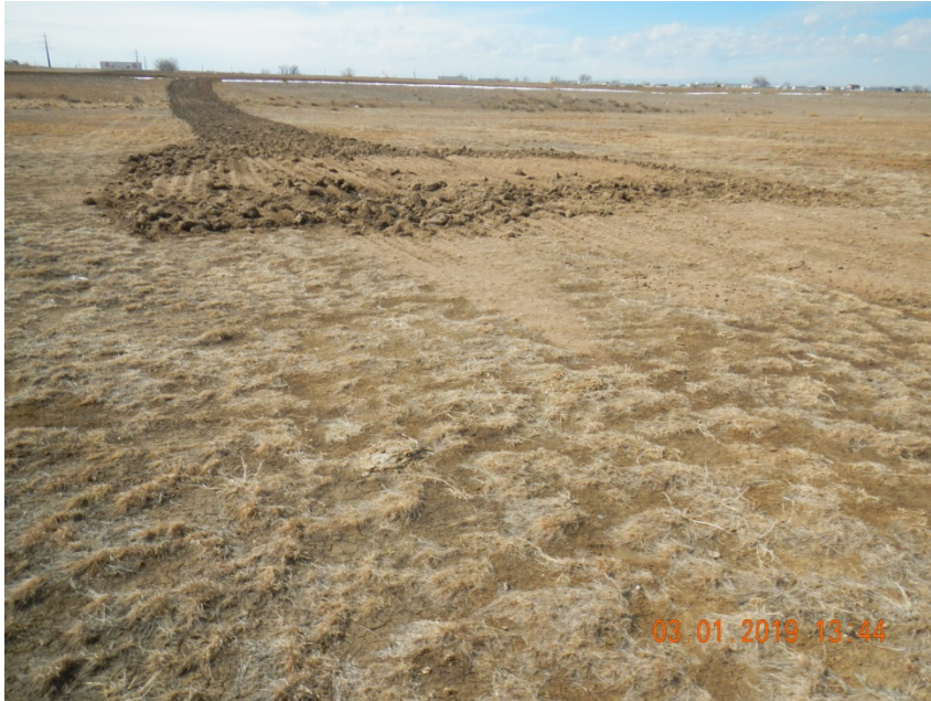
Photo 5. Photo taken from the location, facing West. Appears Operator has recently performed reclamation activities at the location and access road with drill rows observed but no straw crimped mulch. No stormwater BMPs observed at location.
