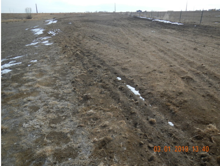
Photo 3. Photo taken from the facility location, facing South. Appears Operator has recently performed reclamation activities with drill rows observed but no straw crimped mulch.
