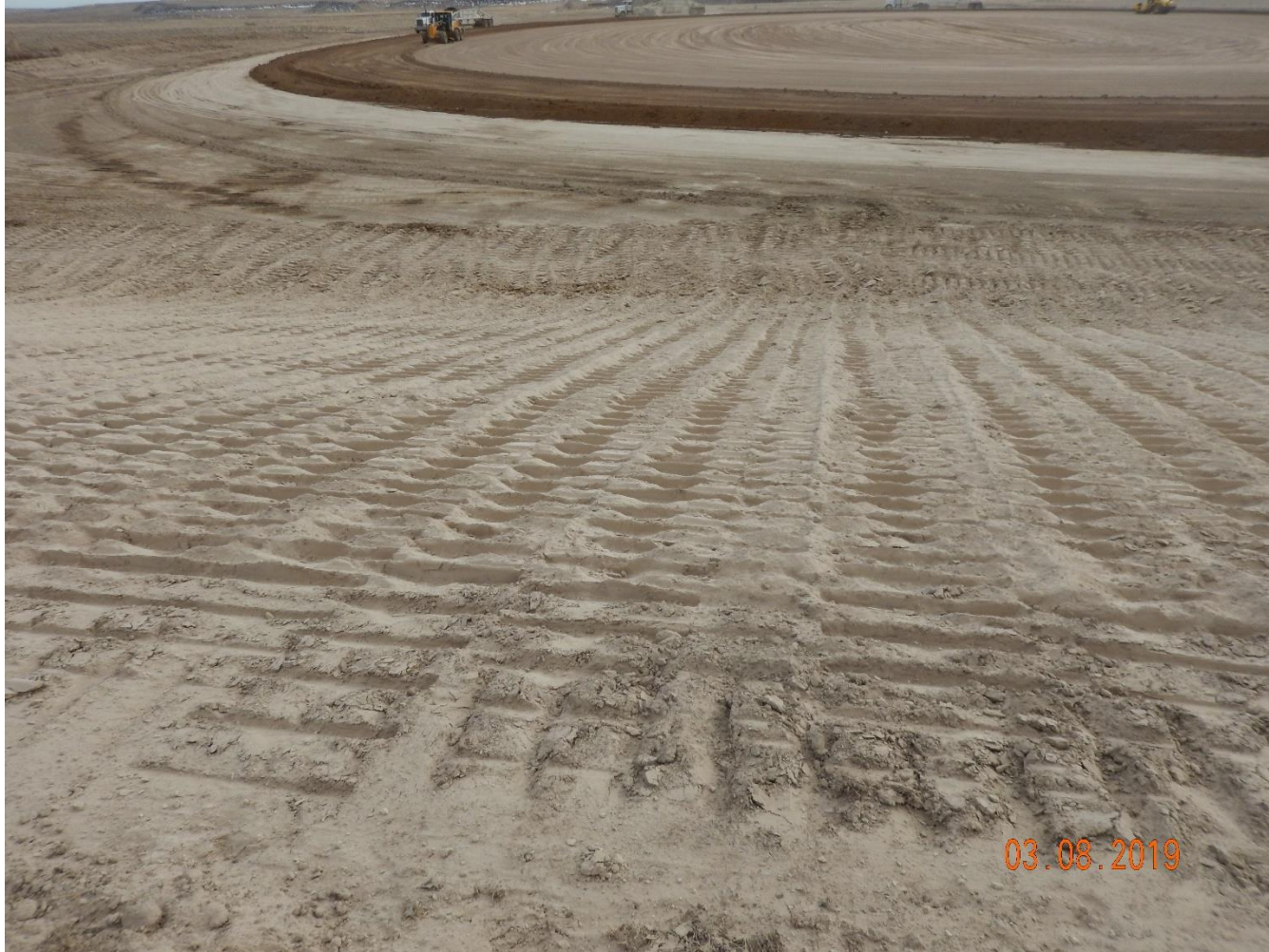
Photo 7: Photo taken from the cut slopes on the northeast corner of the pad. Photo shows areas where operator appears to have sufficiently tracked and stabilized the slopes.
