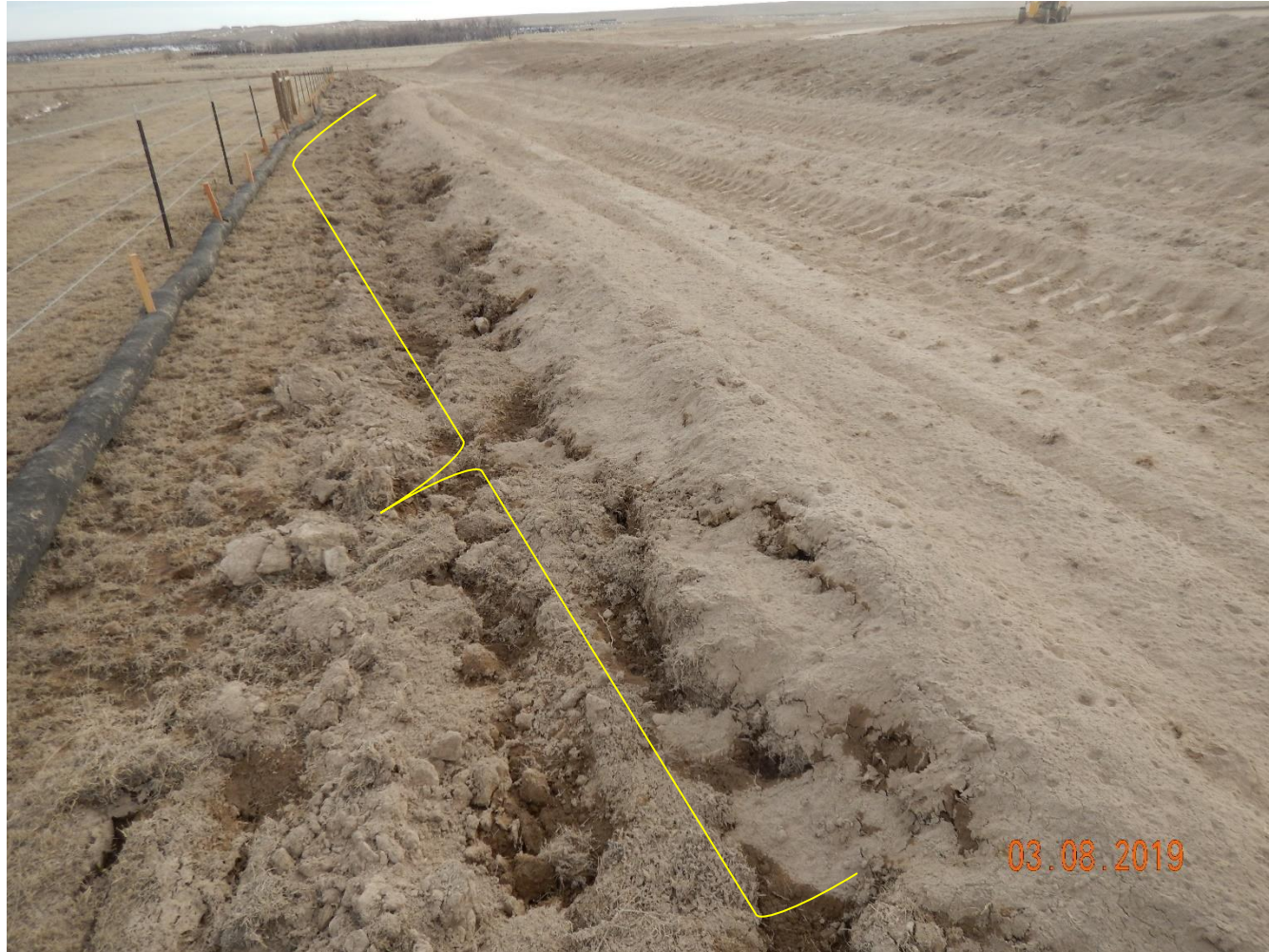
Photo 8: Photo taken from the east end of the location. Photo shows surface roughening (ripping) BMP has filled with sediment and is not longer in proper functioning condition.
