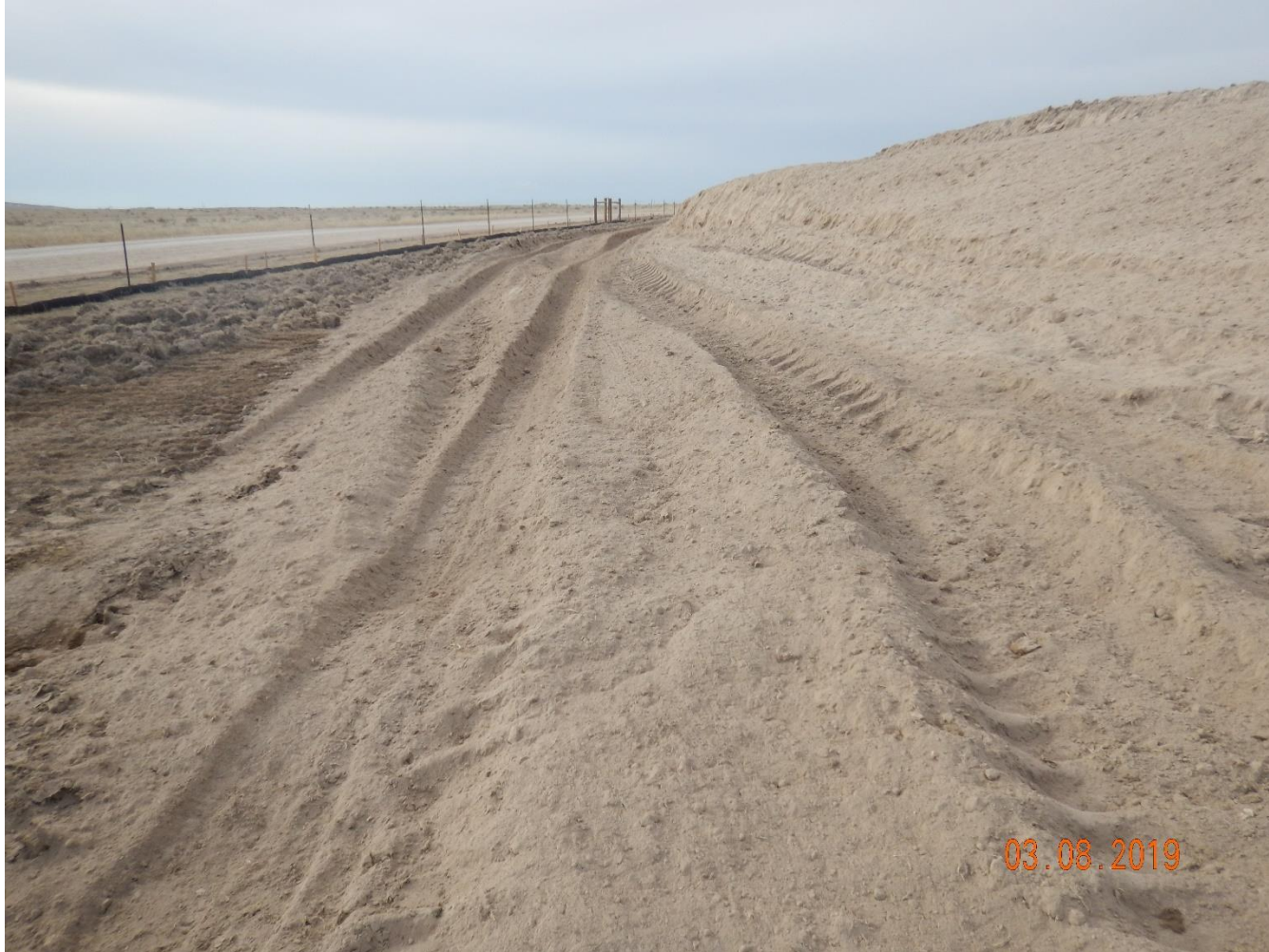
Photo 13: Photo taken from the south end of the location, facing west. Photo shows unstabilized soils on location at risk to erosion degradation.
