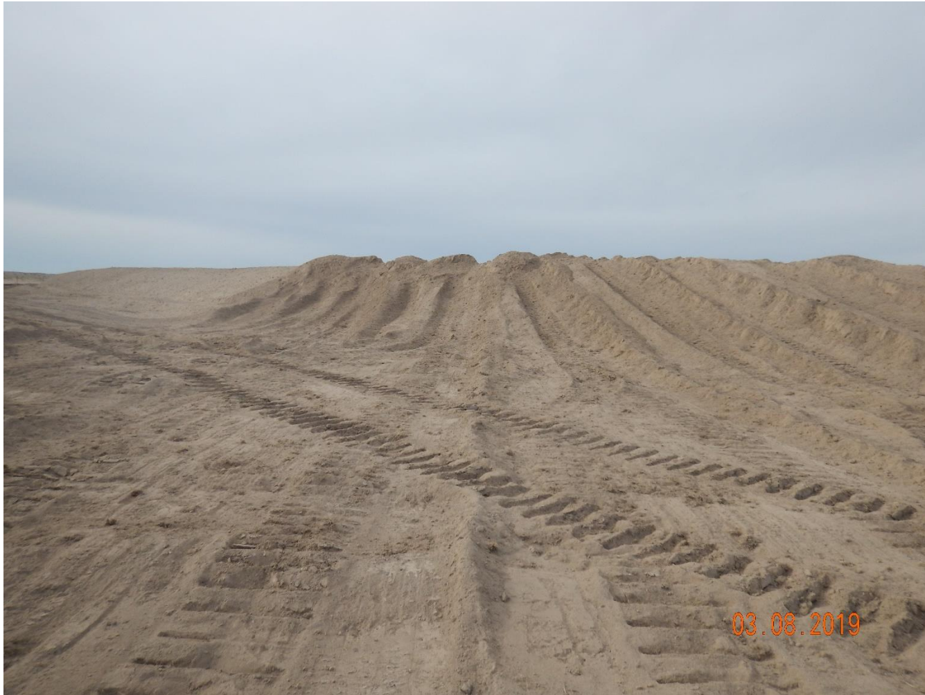
Photo 12: Photo taken from the south end of the location, facing north. Photo shows unstabilized soils on location at risk to erosion degradation
