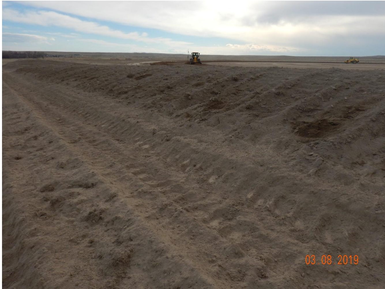
Photo 9: Photo taken from the east end of the location, facing southwest. Photo shows operator has implemented tracking along the slopes. Photo shows BMP has not been sufficiently installed. Soils remain loose material at risk to erosion degradation.
