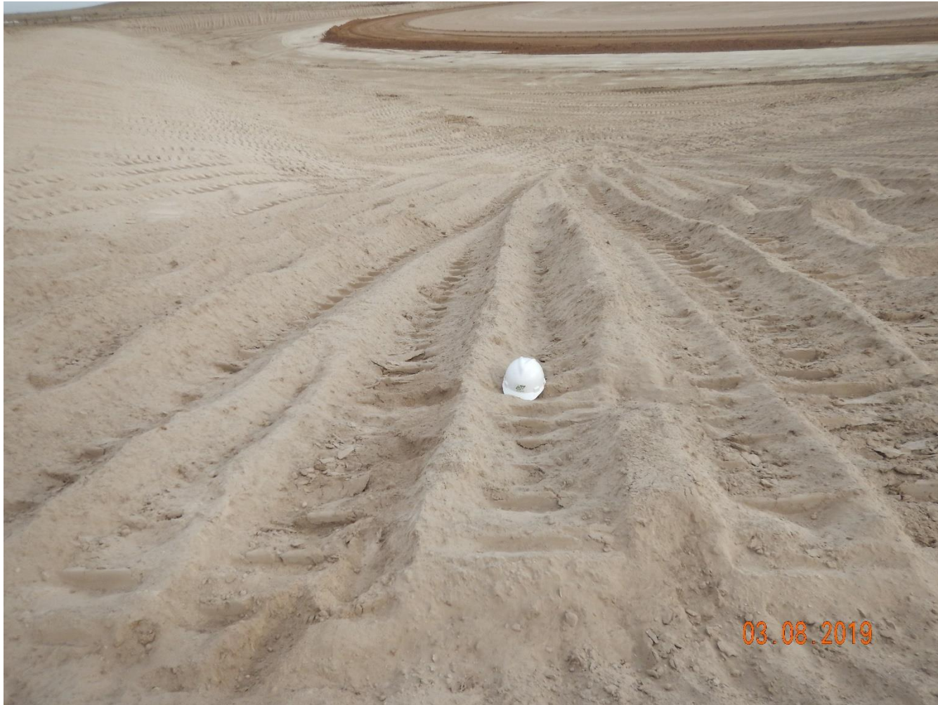
Photo 5: Photo taken from the northwest corner of the pad. Photo shows operator has implemented tracking along the cute slopes. Photo shows BMP has not been sufficiently installed. Soils remain loose material at risk to erosion degradation.
