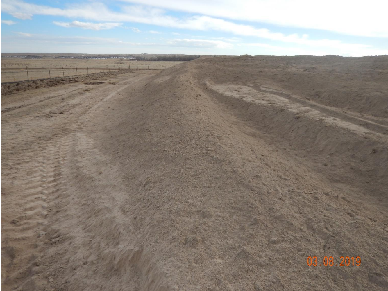
Photo 11: Photo taken from the east end of the location, facing south. Photo shows unstabilized soils on location at risk to erosion degradation.
