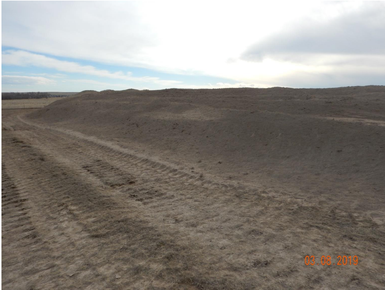
Photo 10: Photo taken from the east end of the location, facing southwest. Photo shows unstabilized soils on location at risk to erosion degradation.
