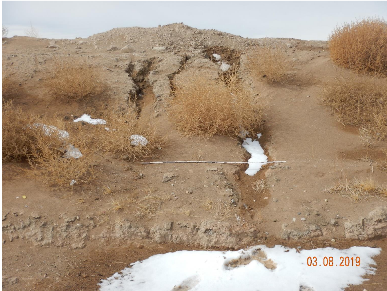
Photo 27: Photo taken from the east end of the pad, facing west. Photo shows slopes are bare and exposed soil, or vegetated by undersirable weedy plant species such as Salsola sp. Slopes have not been sufficiently stabilized. Stormwater erosion and sediment deposition evident. 6 foot measuring stick for reference.
