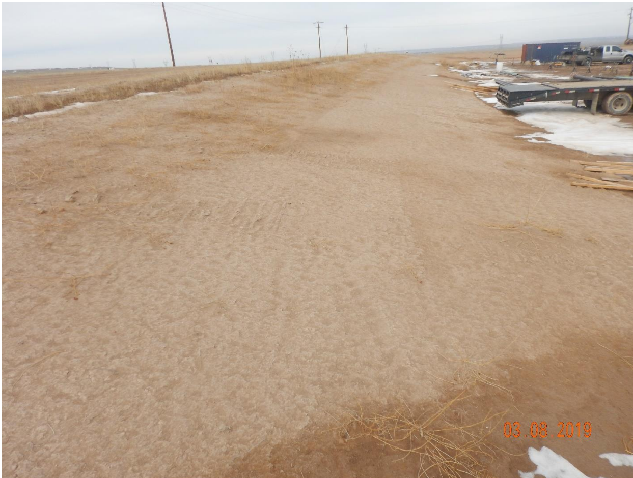
Photo 18: Photo taken from the west end of the location, facing north. Operator appears to have applied a tackier onto the slopes. Cut slopes sufficiently stabilized at time of inspection.
