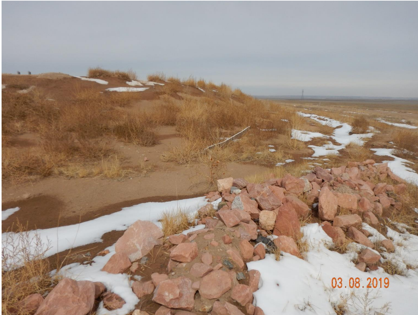
Photo 8: Photo taken from the southeast end of the location, facing north. Photo shows perimeter stormwater ditch on the east end of the location. Ditch does not appear to be sufficient and has filled with sediment. Photo also shows slopes of the pad are bare and exposed soil, or vegetated by undesirable weedy plant species.
