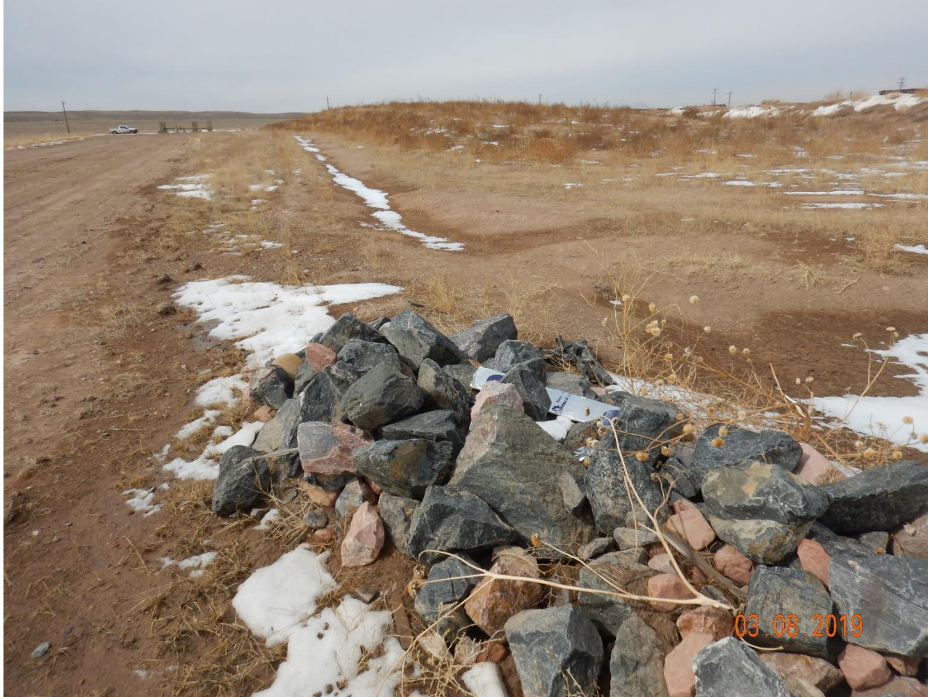
Photo 5: Photo taken from the southeast end of the location, facing west. Photo shows perimeter stormwater ditch on the south end of the location, and the topsoil stockpile. Ditch does not appear to be sufficient and has filled with sediment.
