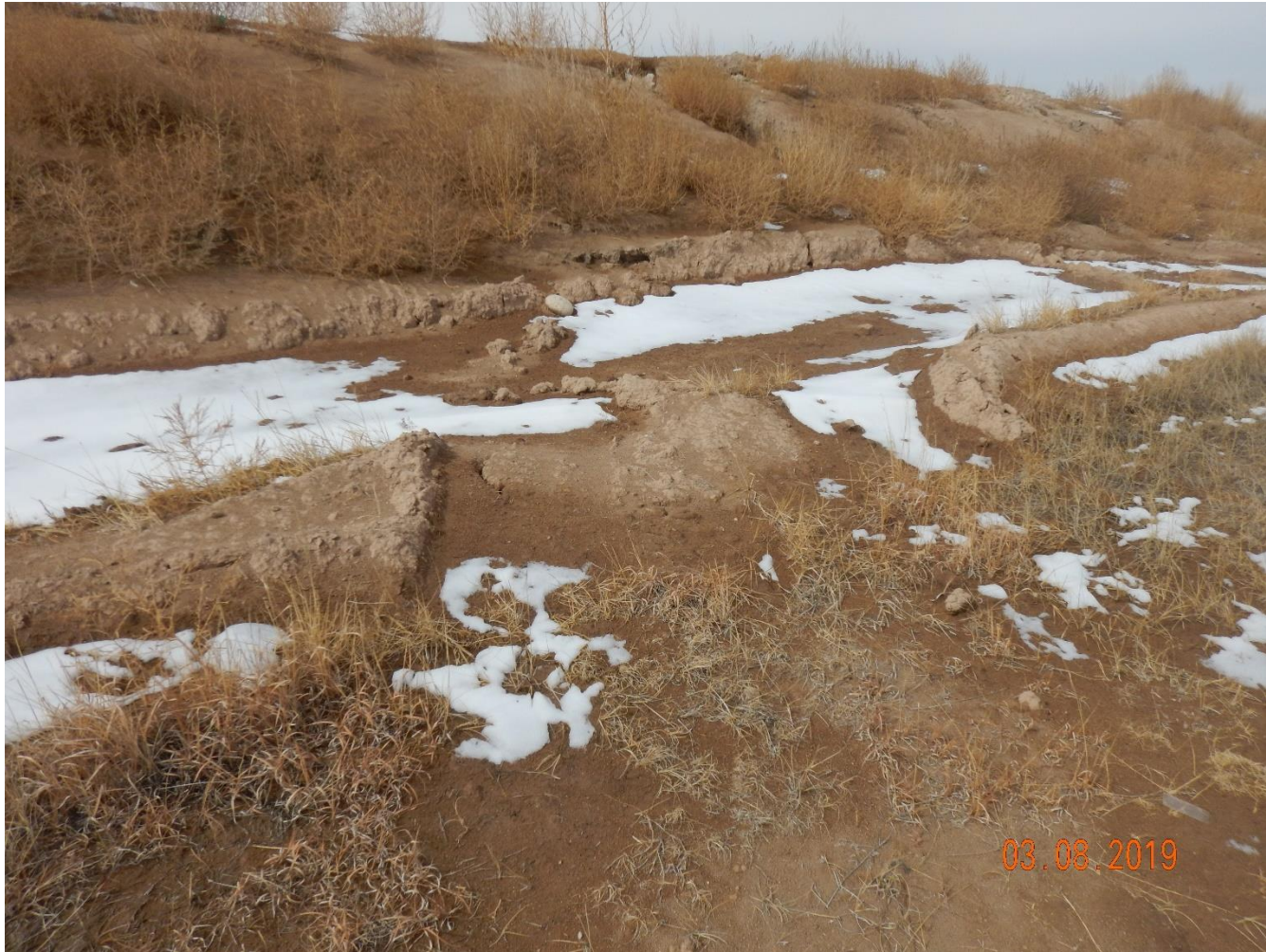
Photo 34: Photo taken from the ditch on the east end of the location. Photo shows a vehicle appears to have traveled over and damaged the ditch/berm. BMP no longer in proper functioning condition.
