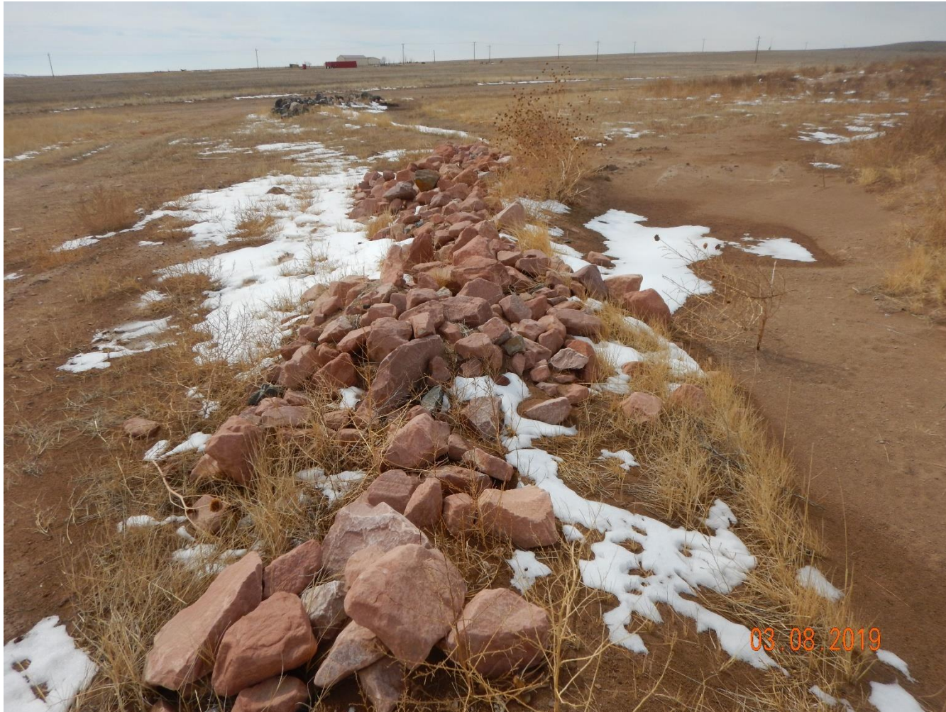
Photo 9: Photo taken from the southeast end of the location, facing south. Photo shows perimeter stormwater ditch on the east end of the location. Ditch does not appear to be sufficient and has filled with sediment.
