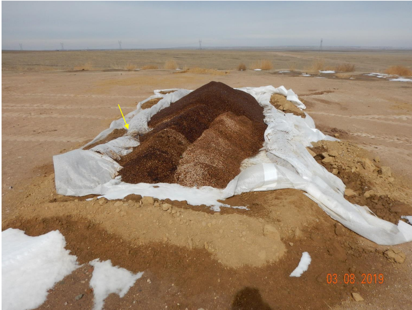
Photo 41: Photo taken from the northeast corner of the pad. Photo shows Operator is storing contaminated soils on the northeast corner of the pad. Containment BMPs are insufficient as pollutant discharge from the contaminated soils is evident.
