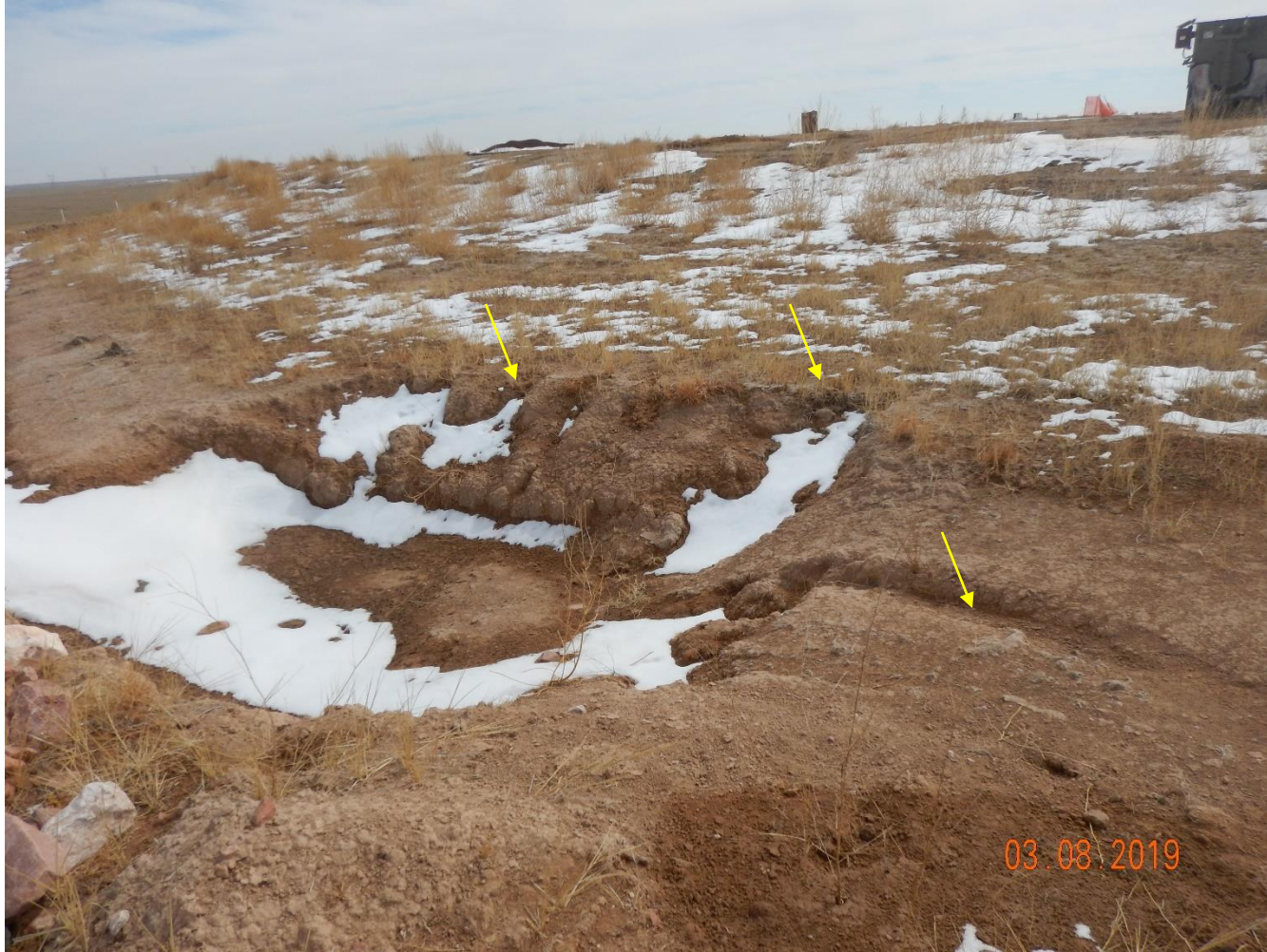
Photo 40: See comments under photo 27. In addition It does not appear that the perimeter stormwater and erosion controls installed on location are sufficient to mitigate stormwater runoff from the 11 acre disturbance; The two (2) sediment traps on the northeast and northern ends of the location also do not appear to be sufficient in size for the location.
