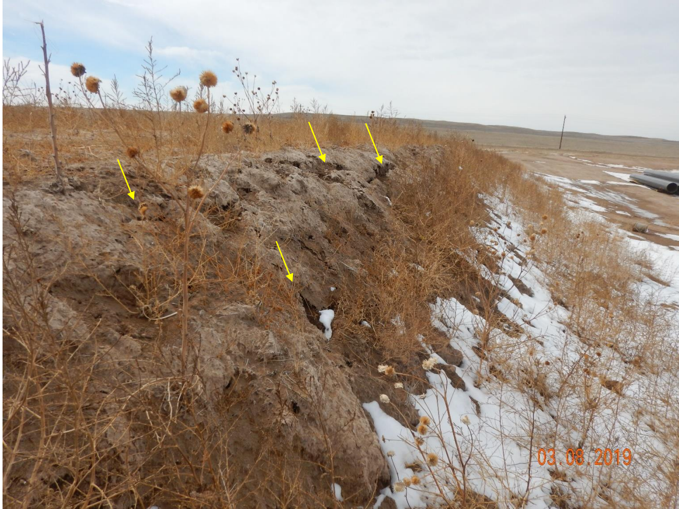
Photo 20: Photo taken from the north facing slope of the topsoil stockpile. Operator does not appear to have constructed the stockpile with an appropriate grade. Photo shows slopes do not appear to be sufficiently stabilized. Erosion degradation evident.
