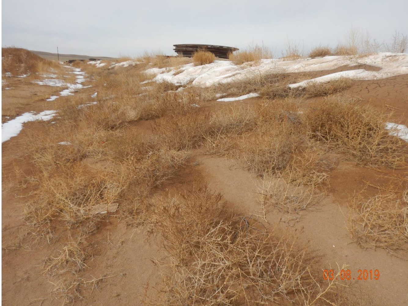
Photo 24: Photo taken from the slopes on the south end of the pad. Photo shows slopes are bare and exposed soil, or vegetated by undersirable weedy plant species such as Salsola sp. Slopes have not been sufficiently stabilized. Stormwater erosion and sediment deposition evident.
