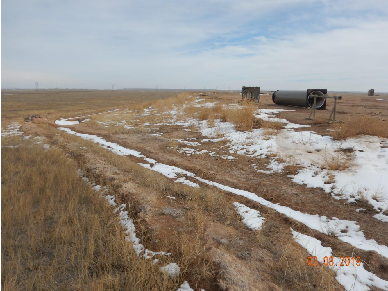
Photo 10: Photo taken from north end of the location, facing southeast. Photo shows slopes of the pad and the perimeter stormwater ditch. Slopes of the pad are bare and exposed soil, or vegetated by undesirable weedy plant species.
