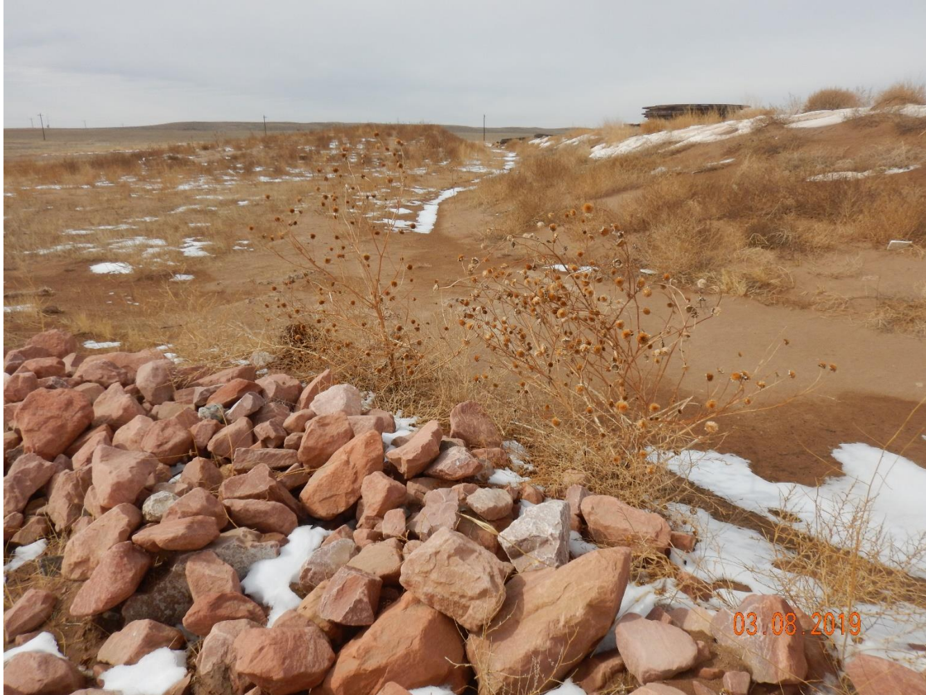
Photo 7: Photo taken from the southeast end of the location, facing west. Photo shows stormwater ditch between pad and the topsoil stockpile. Ditch does not appear to be sufficient and has filled with sediment.
