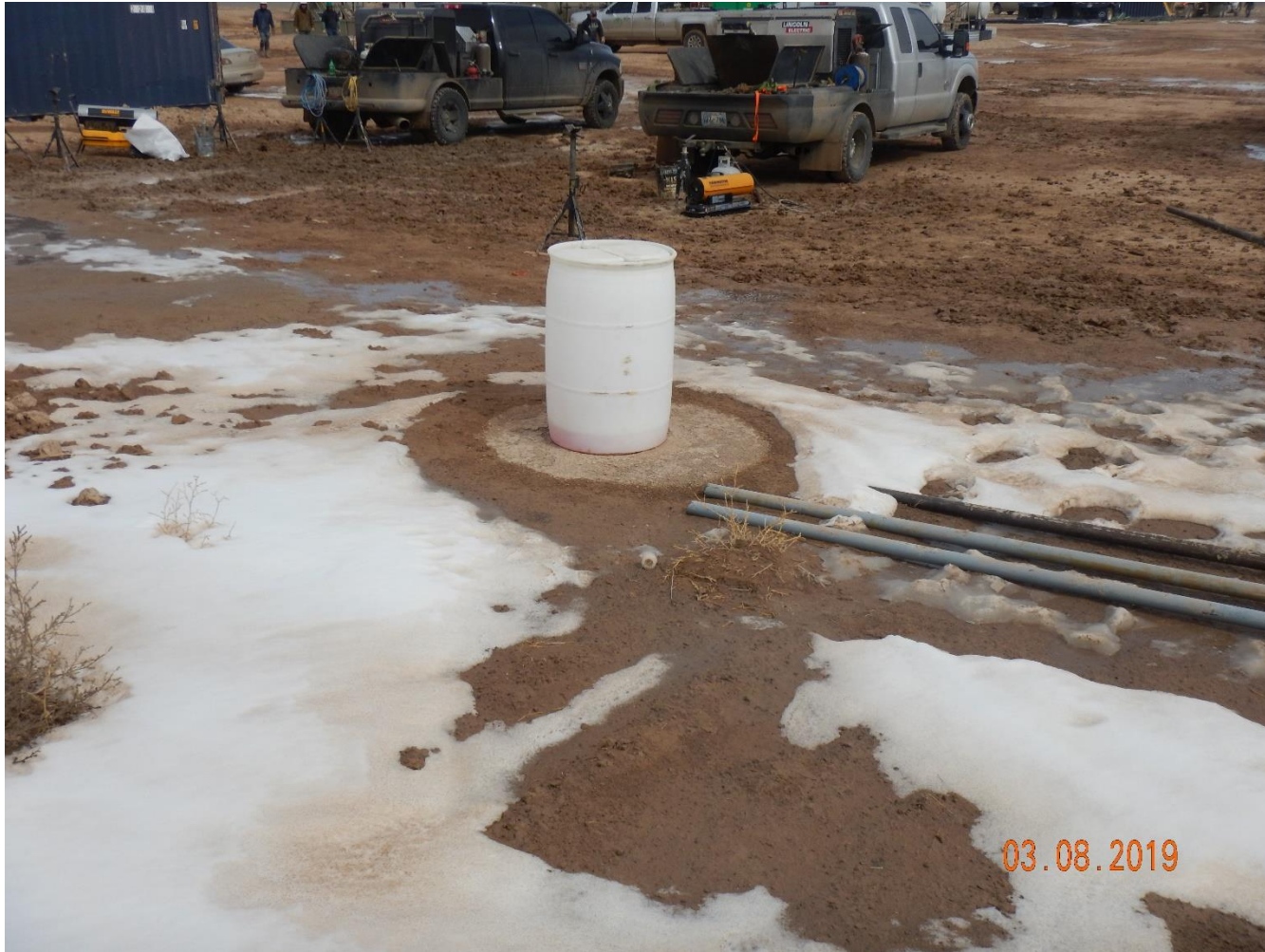
Photo 46: Photo taken from the west end of the pad. Photo shows a barrel being stored directly upon the surface of the soil. This is not proper materials management.
