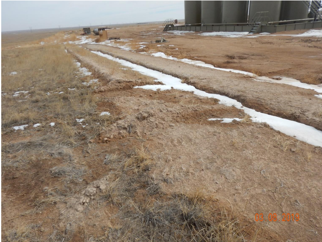
Photo 12: Photo taken from the north end of the location, facing east. Photo shows areas of the ditch where vehicles were operated over the BMP. This is not advised.
