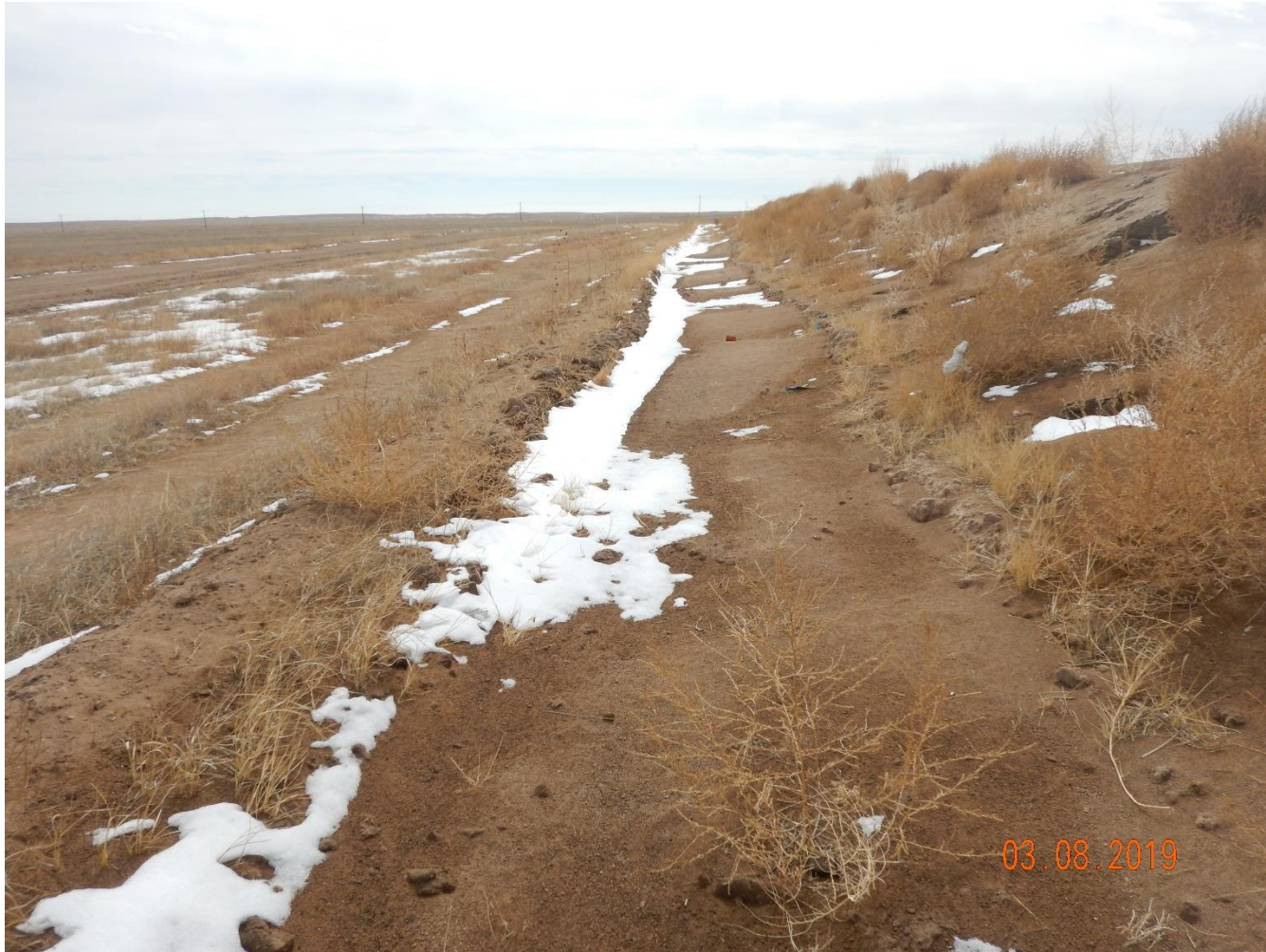
Photo 32: Photo taken from the east end of the location, facing south. Photo shows ditch has filled with sediment and is not longer in proper functioning condition.
