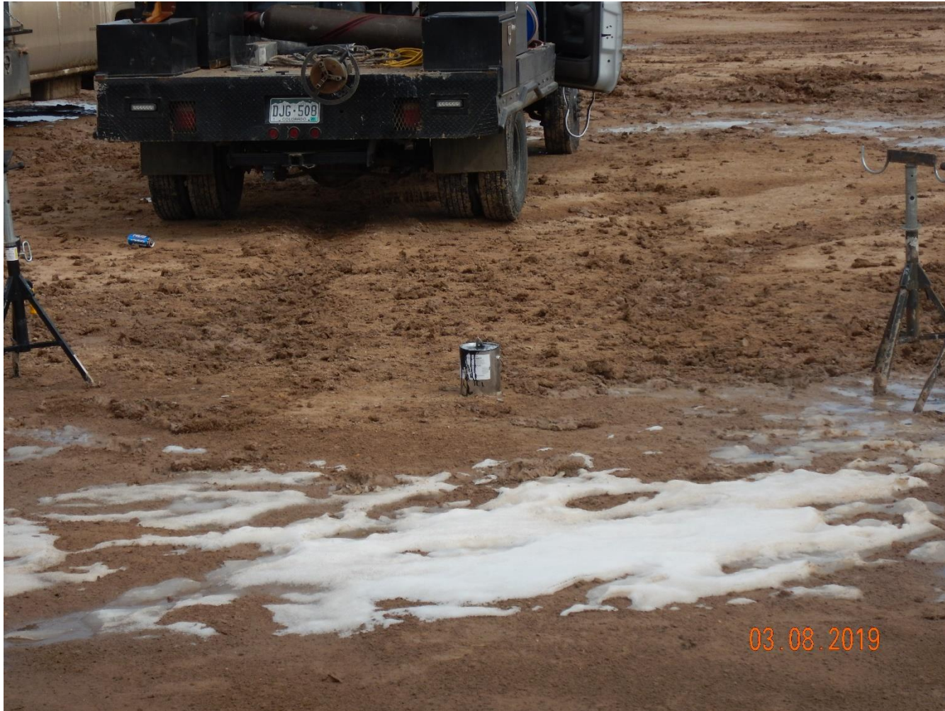
Photo 47: Photo taken from the west end of the pad. Photo shows what appears to be a paint can being stored directly upon the surface of the soil. This is not proper materials management.
