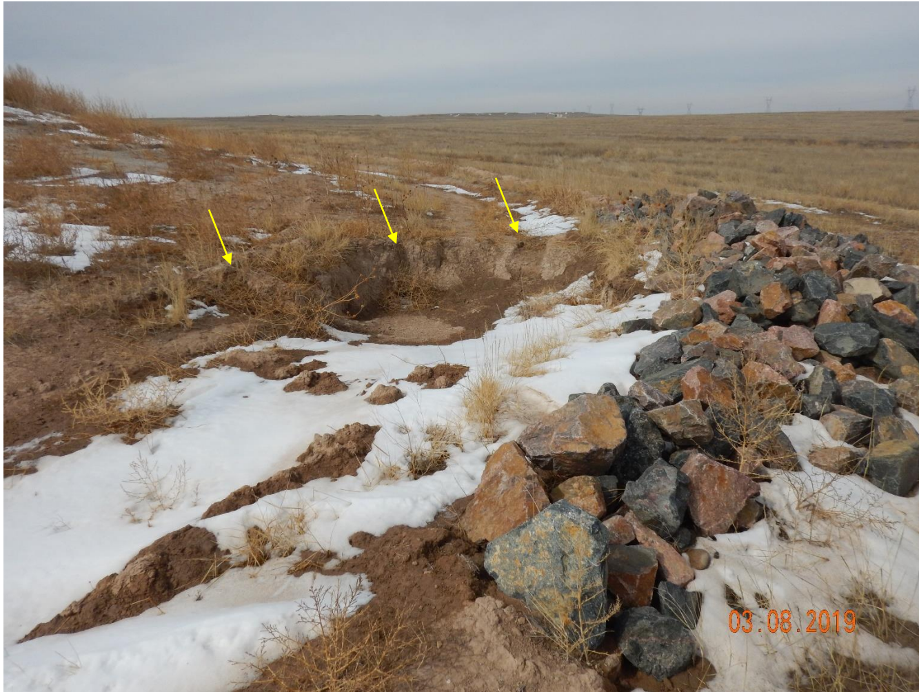
Photo 37: Photo taken from the sediment trap on the northeast corner of the location. BMP does not appear to have been constructed in accordance with good engineering practices; insufficient inlet and slope protection. Stormwater has incised the ditch at the inlets of the sediment traps. Slopes of the traps do not appear to have been constructed at an advisable grade in accordance with good engineering practices; stormwater erosion degradation evident along the slopes of the sediment traps.
