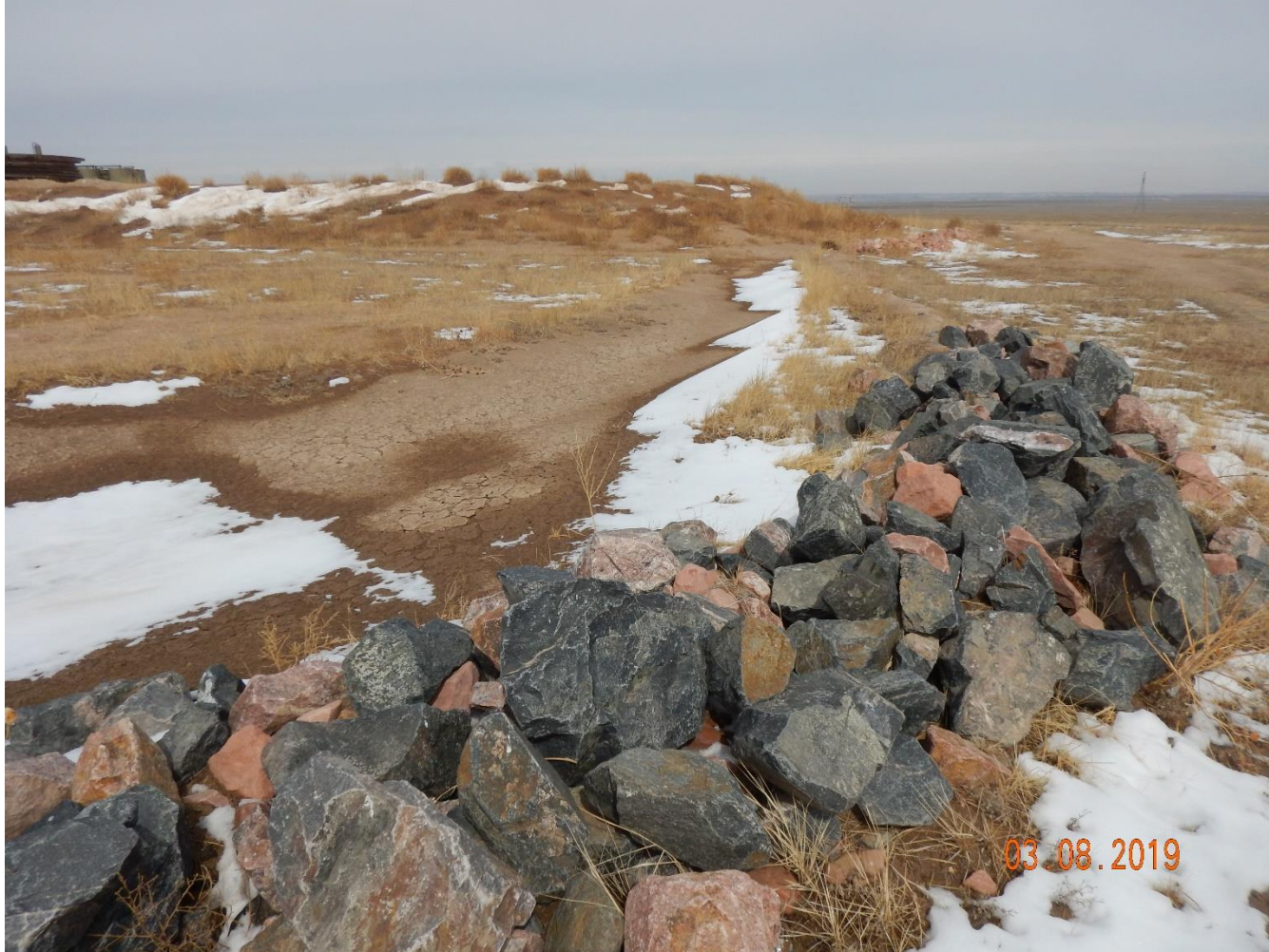
Photo 6: Photo taken from the southeast end of the location, facing north. Photo shows perimeter stormwater ditch on the east end of the location. Ditch does not appear to be sufficient and has filled with sediment.
