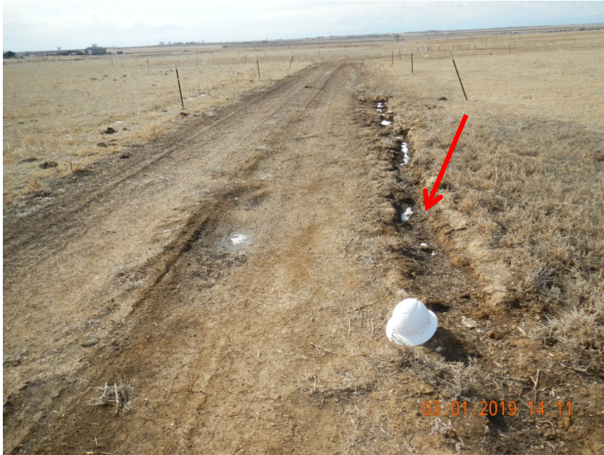
Photo 3. Photo taken from the access road, facing West. Photo depicts erosion observed on the north side of the road.
