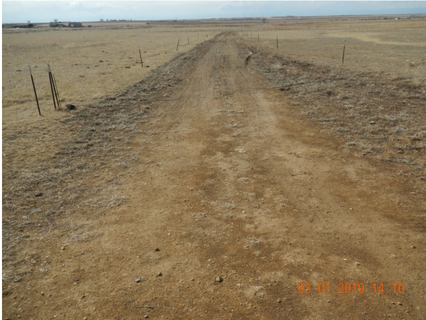
Photo 1. Photo taken from the access road off CR 55, facing West. Photo depicts the access road remains on location, the gravel has not been removed and has not been re-contoured or re-graded and decompacted to meet the adjacent terrain.
