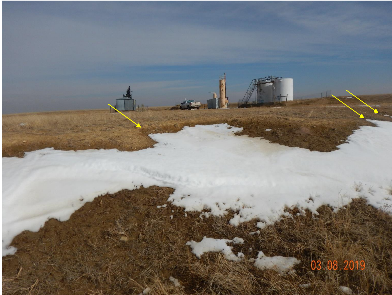
Photo 16: PhoPhoto taken from the south end of the location, facing northeast. Previous inspections documented erosion degradation on the location and required operator to implement BMPs in accordance with 1002.f. Photo shows erosion degradation remains, no BMPs have been installed or maintained.
