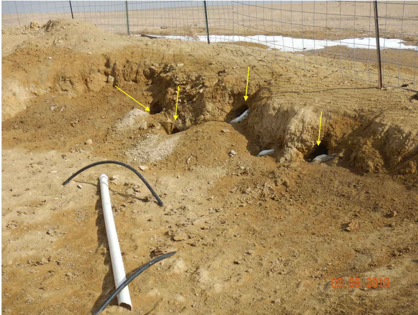
Photo 24: Photo taken from the pit, facing northeast. Photo shows wildlife have burrowed into the walls of the pit compromising the integrity of the pit walls.
