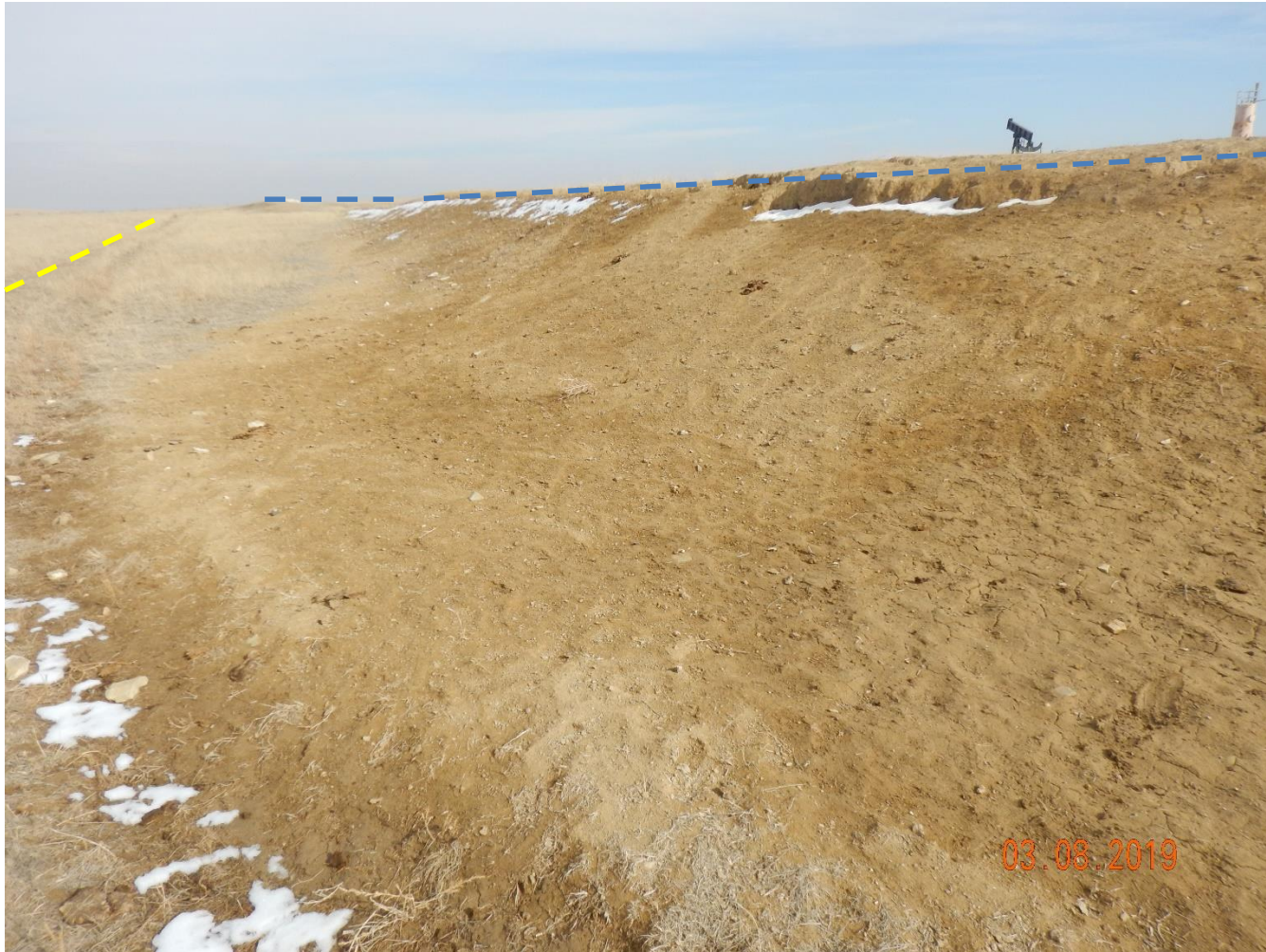
Photo 13: Photo taken from the southwest corner of the location, facing northeast. Previous inspections documented slopes on location remain predominantly bare and exposed soil with stormwater erosion degradation evident. Slopes remains bare and erosion degradation remains evident.
