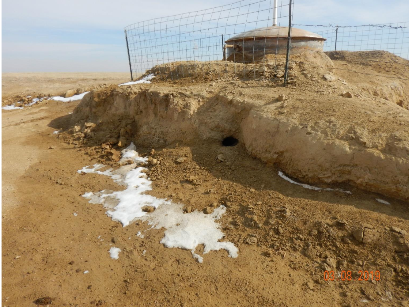
Photo 22: Photo taken from the west end of the unpermitted pit, facing northeast. Photo shows wildlife have burrowed into the walls of the pit compromising the integrity of the pit walls.
