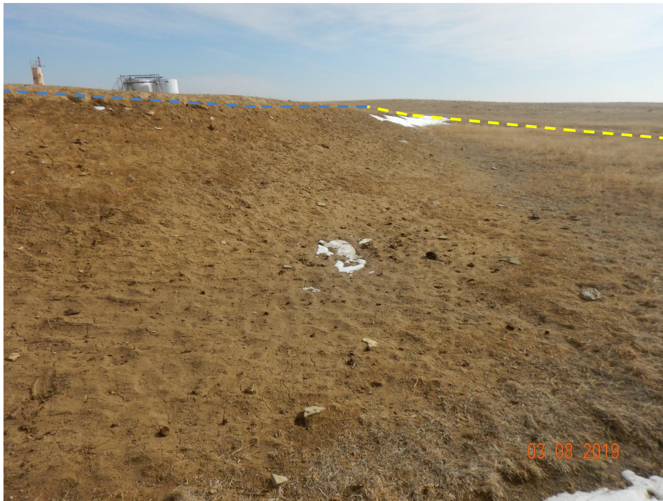
Photo 14: Photo taken from the southwest corner of the location, facing east. Previous inspections documented slopes on location remain predominantly bare and exposed soil with stormwater erosion degradation evident. Slopes remains bare and erosion degradation remains evident.
