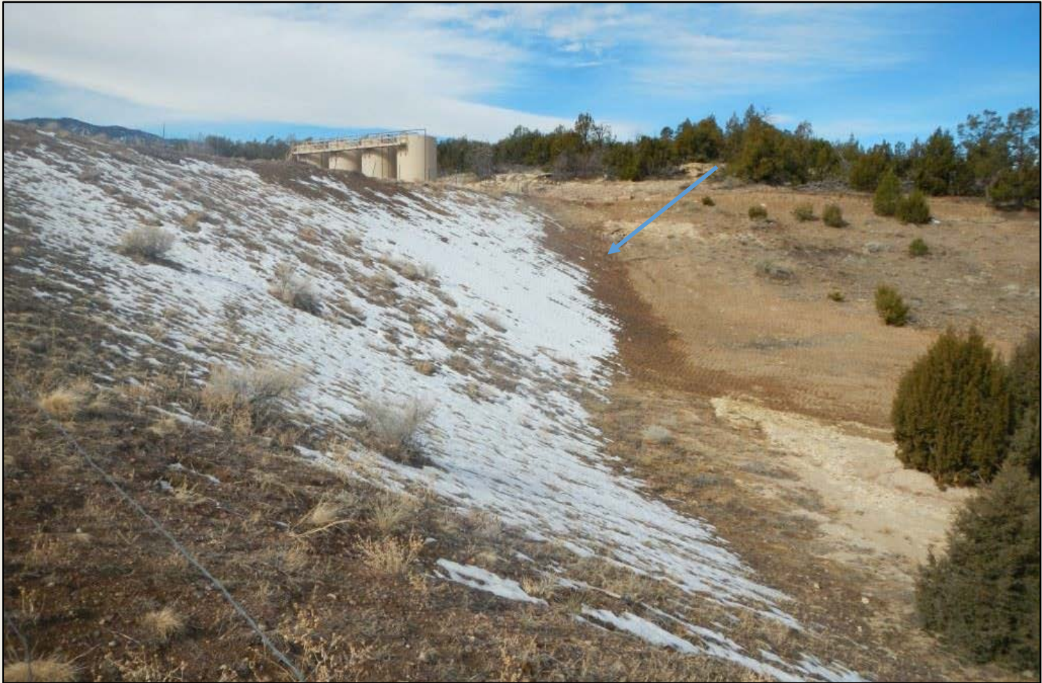
Photo 1. View of the northeastern project area from the access road facing northward. Erosion is occurring in area where arrow is pointing, and long term erosion control is needed in this area.
