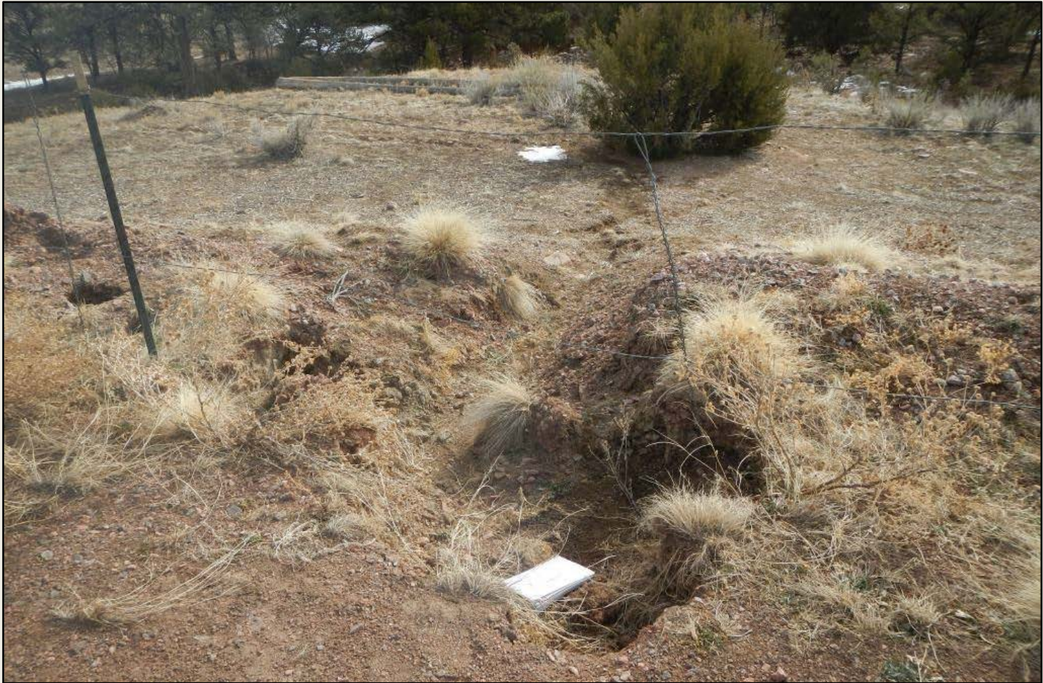
Photo 4. View of erosional channel approximately 3 feet wide and 2 feet deep, forming in the eastern project area where concentrated stormwater flows off of the well pad.
