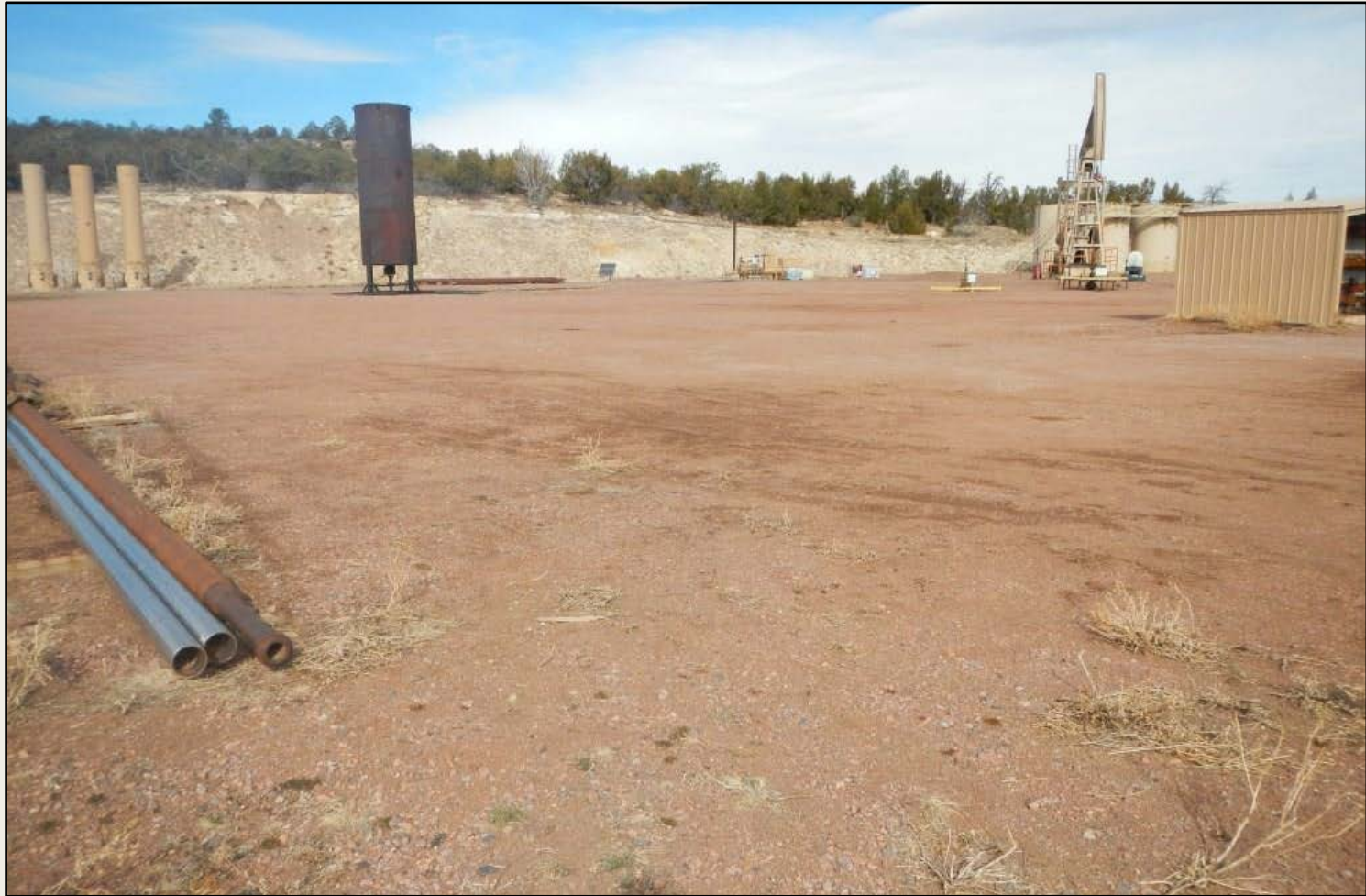
Photo 3. View of the project area from the southeastern corner facing center. Interim reclamation needs to be conducted as large portions of the well pad do not appear needed for existing production operations. Date of first production was November 22, 2012. Therefore interim reclamation should have been conducted by May 22, 2013.
