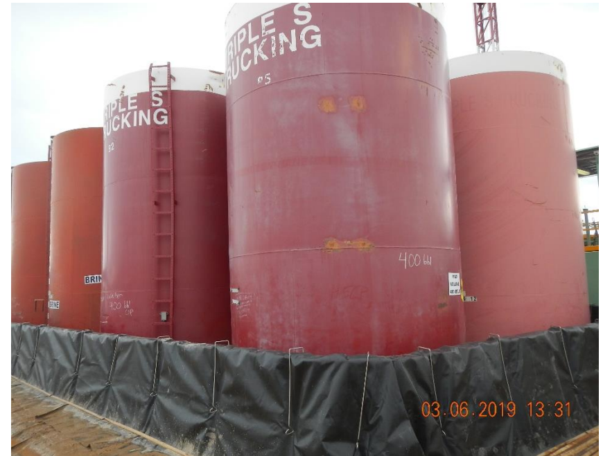
Lined secondary containment berm for fresh water/brine ASTs.
