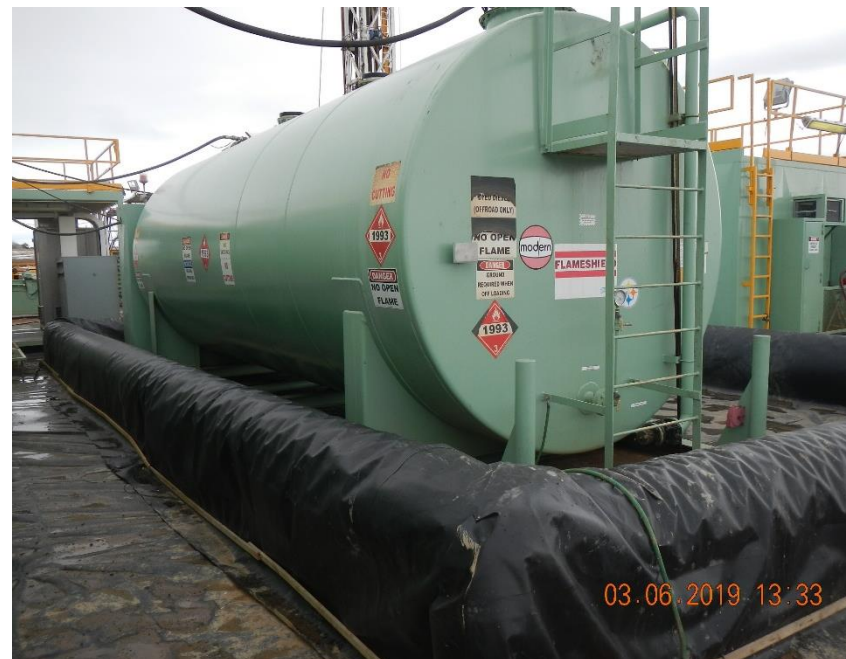
Diesel fuel container with secondary containment.
