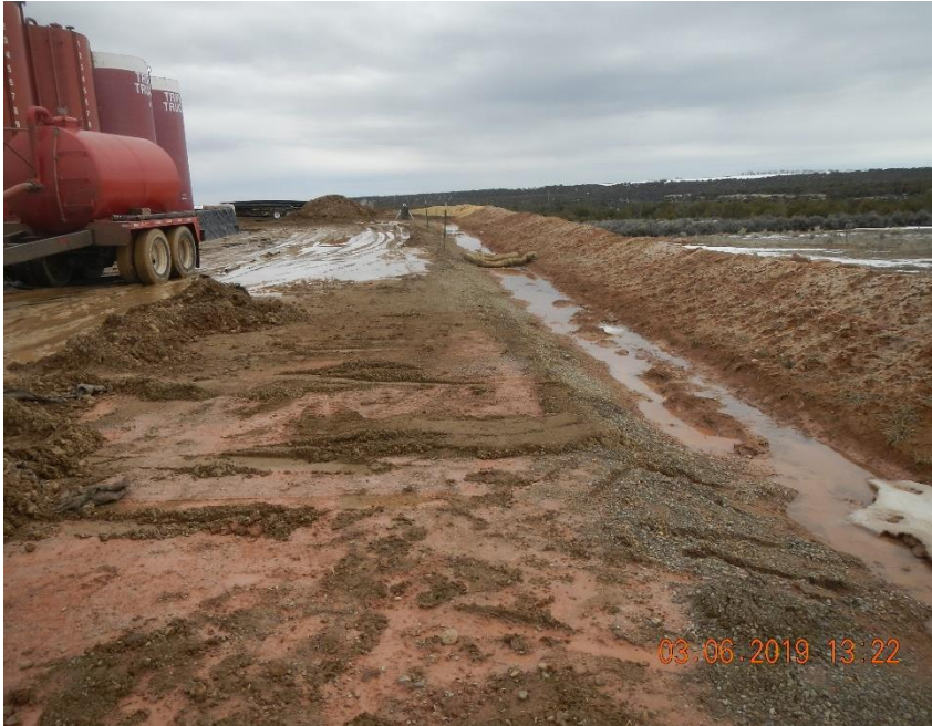
Terminus of drilling fluid release in perimeter ditch along N edge of location.
