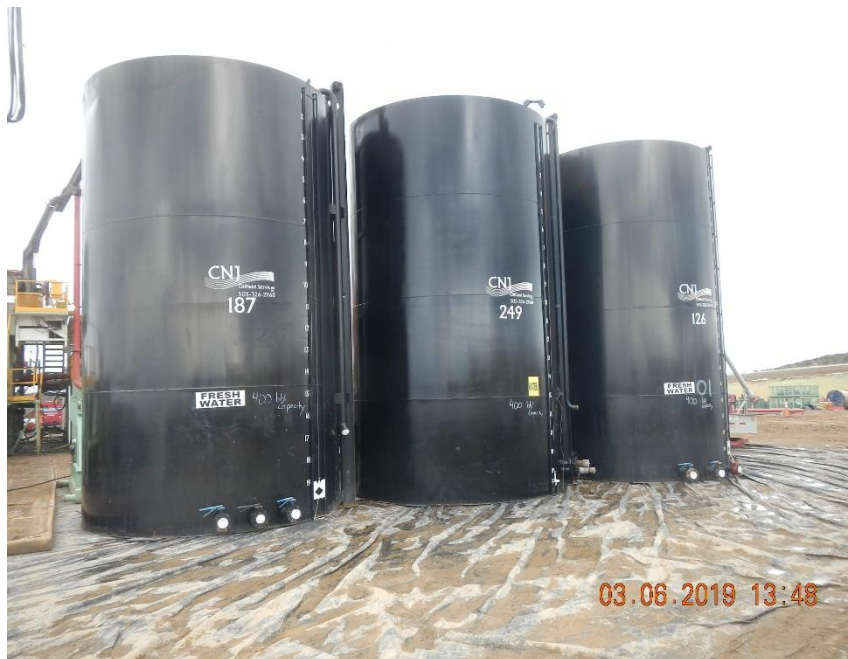
Three 400 bbl. ASTs labeled fresh water.
