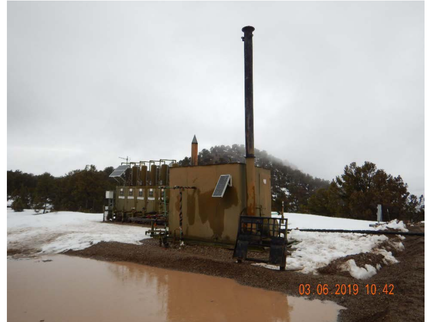
Photo #4 – View of heated horizontal separator (foreground) and heated vertical separators (background), located west of frac tank. Note that heated horizontal separator in foreground lacks bird protection.
