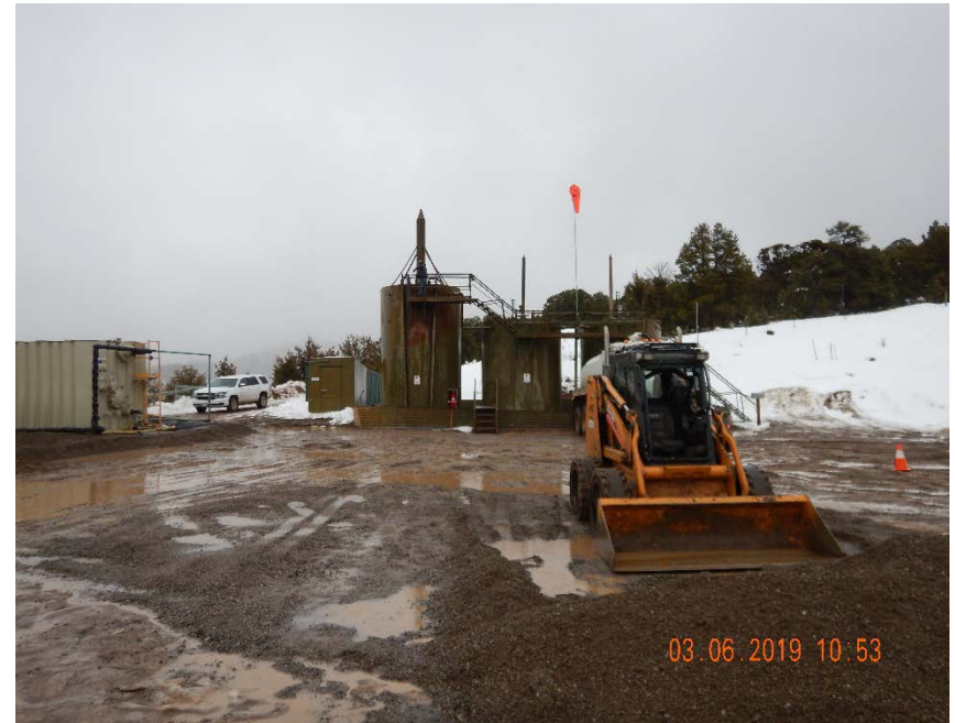
Photo #2 – View of existing tank battery from wellhead, looking east. Note presence of frac tank on left side of photo and puddles of stormwater throughout pad.
