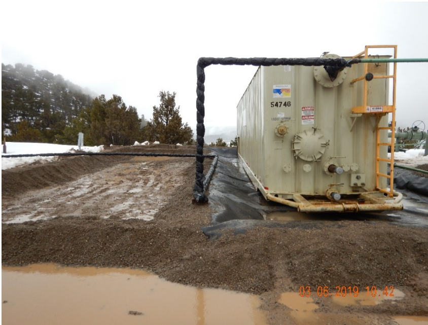
Photo #3 – View of temporary tank battery from south. Note that liner has been installed beneath frac tank but earthen berm lacks compaction. Berm capacity may not be sufficient to contain contents of frac tank plus freeboard, per 605.a.(4).
