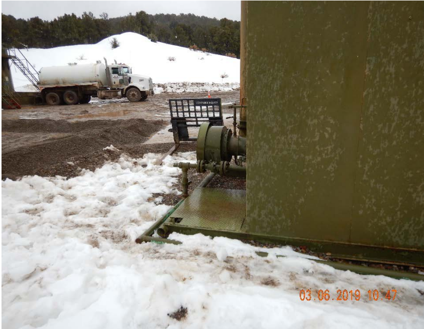
Photo #5 – View of vertical heated separator array from north. Distance from this point on separator to frac tank was measured to be 60' on inspection date.
