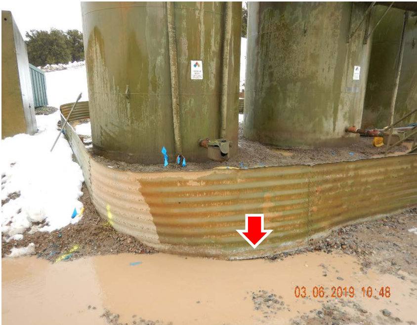
Photo #7 – View of existing tank battery containment device at northwest corner. Note that base of metal ring is visible (red arrow).
