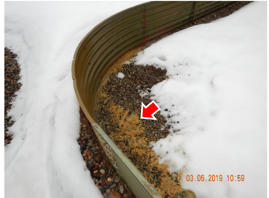
Photo #8 – Fluid accumulation within existing tank battery containment (red arrow). Work to delineate and remediate impacts within existing tank battery is proceeding under Remediation Project #12674.
