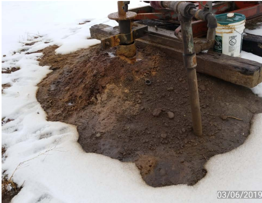
Photo 3. Oil staining on ground at wellhead.
