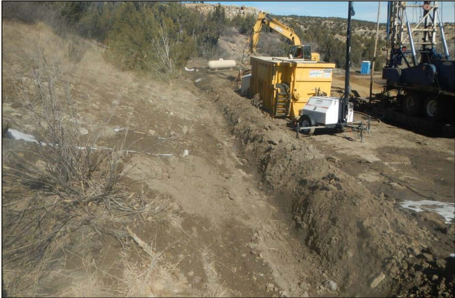
Photo 6. View of the western project area from the southwestern edge facing northward. Berms are not properly compacted and ditches are not stabilized. Loose soil within ditch bed will rapidly wash down gradient.
