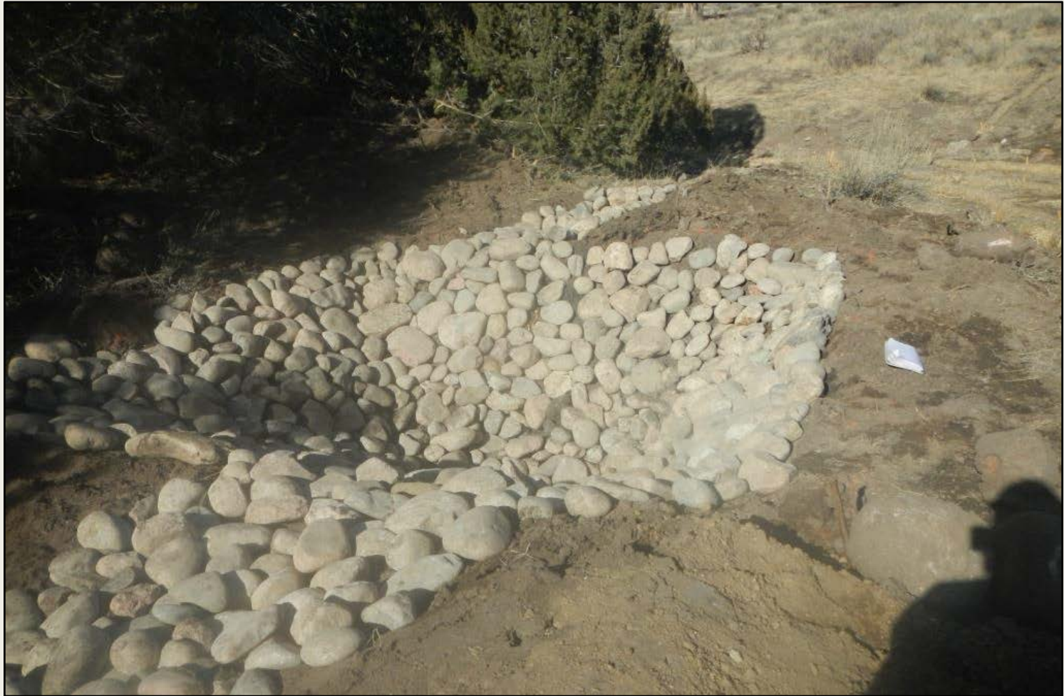
Photo 10. View of sediment trap within the northern project area. See comments on Photo 5.
