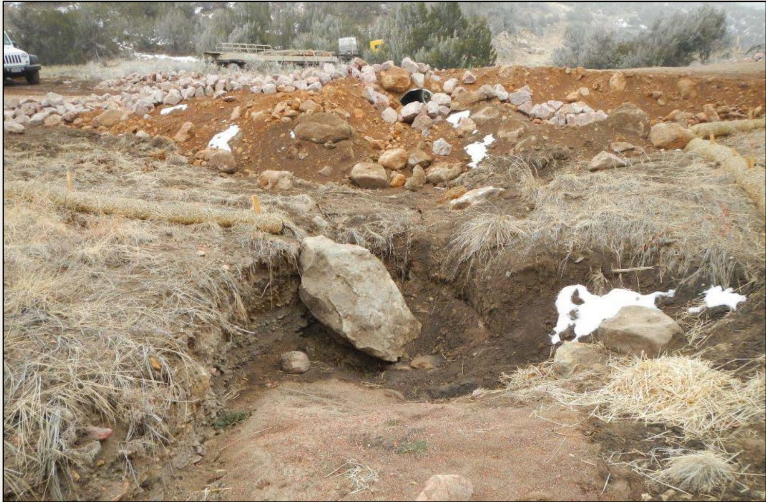
Photo 13. View of culvert outlet facing southward, upstream. Culvert outlet is partially blocked with rock and soil. Head-cut that is approximately 3 feet tall and 3.5 feet wide will need stabilization as concentrated stormwater flows from the culvert will likely accelerate erosion. Stream crossing has not been properly constructed see Photo 12.
