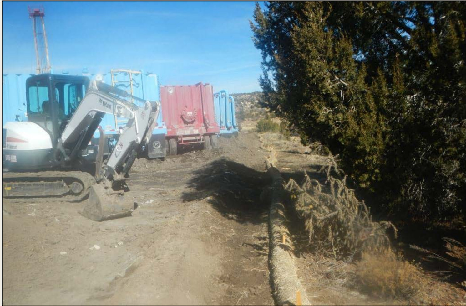
Photo 4. View of the eastern project area from the southeastern corner facing southward. Berms appear to be comprised of topsoil and are not properly installed. Controls in place do not appear to be sufficient to control stormwater from the location.
