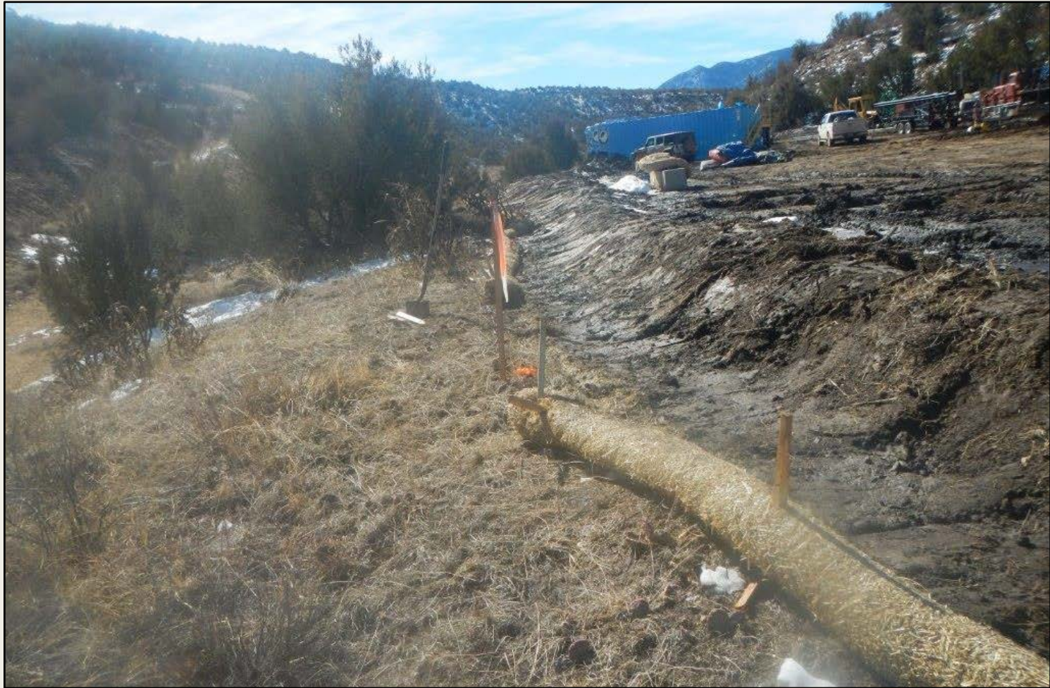
Photo 2. View of the eastern portion of the project area from the northeastern corner facing southward. Wattles are not properly installed due to lack of trenching, and gaps along the boundary remain.
