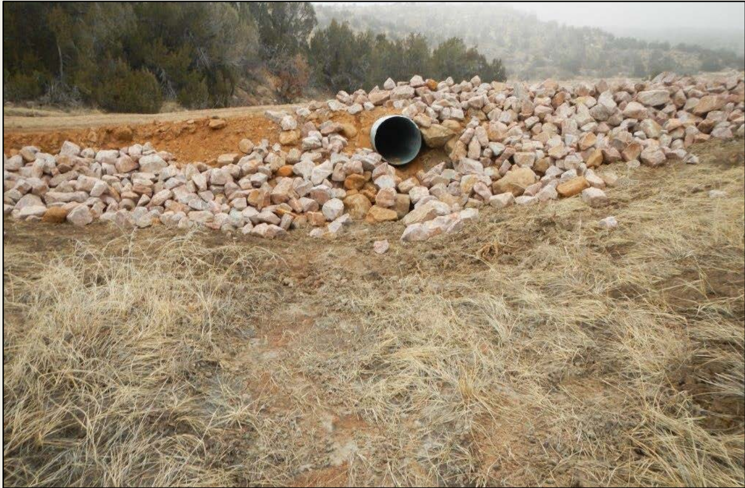
Photo 12. View of culvert inlet facing northward, downstream. Culvert is approximately 3 feet above ground elevation and not properly constructed for a stream crossing.
