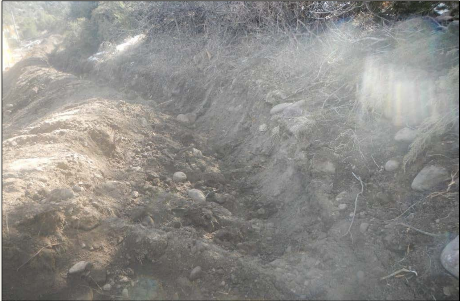
Photo 8. View of ditch within the western project area. Cut bank, berms and ditch bottom are not stabilized or properly installed.
