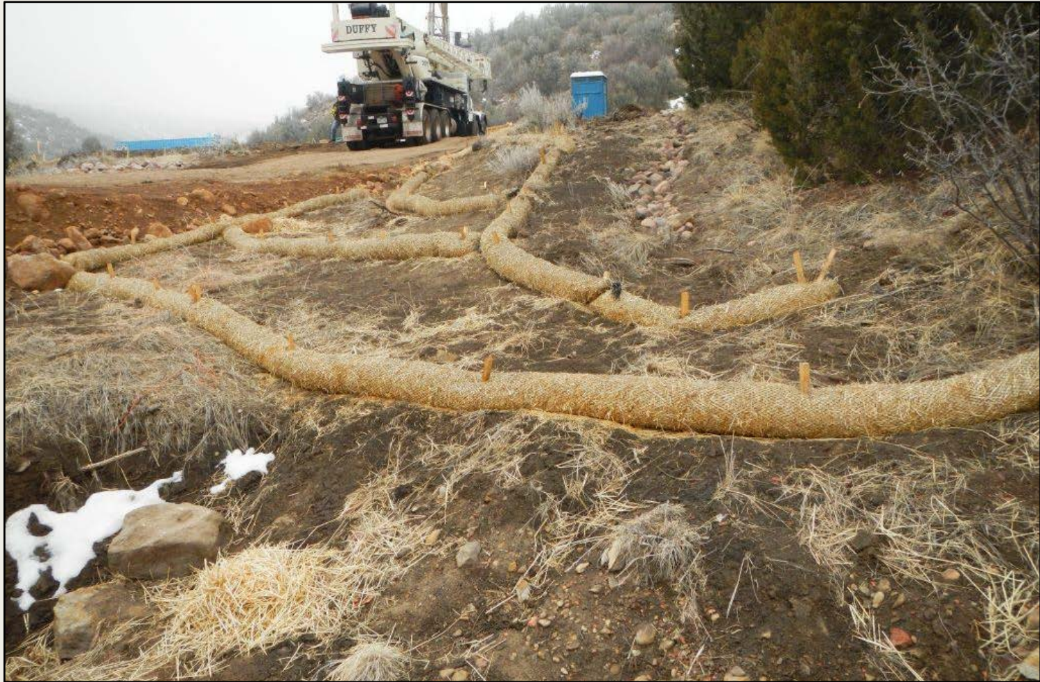
Photo 14. View of wattles and straw placed in the northern project area. Wattles and BMP are not properly installed.
