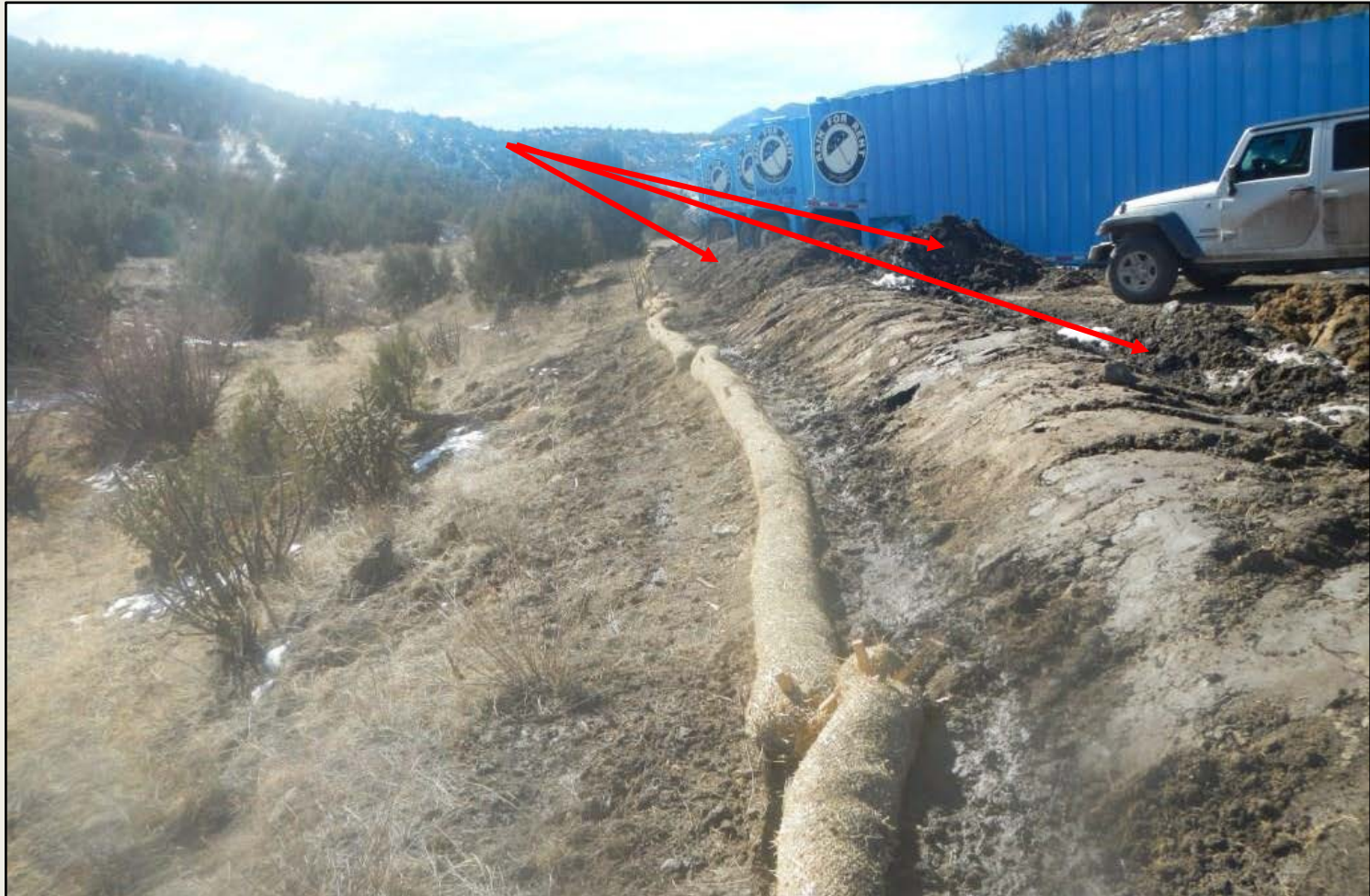
Photo 3. View of the southeastern edge of the project area from the eastern edge facing southward. Wattles are not properly placed as loose soil down slope from wattles needs stabilization, and wattles are not properly installed (see Photo 2). Arrows indicate improperly salvaged and protected topsoil.
