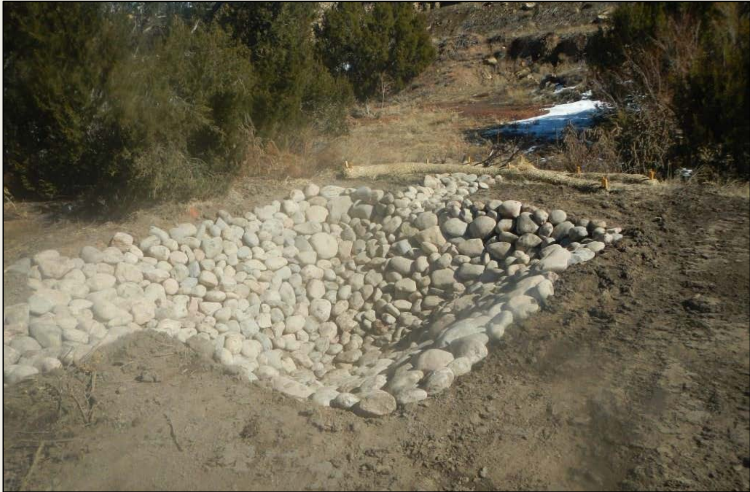
Photo 5. View of sediment trap run-on control, in the southeastern project area; recently redesigned. However, sediment trap has not been properly constructed due to the use of rounded cobble which is not considered a good engineering practice. It is expected that stormwater flows will undermine the cobble material. Angular rock and geotextile fabric should be used per good engineering practices.
