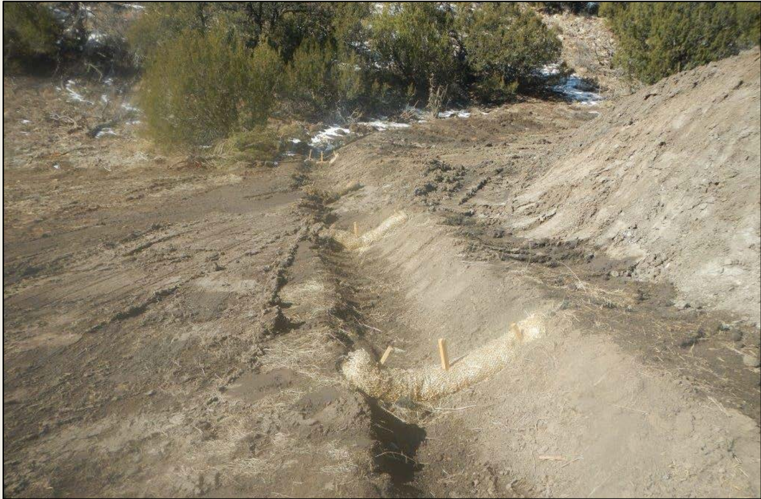
Photo 7. View of southern project area from the southeastern corner facing westward. Check dams not properly installed, or with the best engineering materials. Loose material remains in the ditch.
