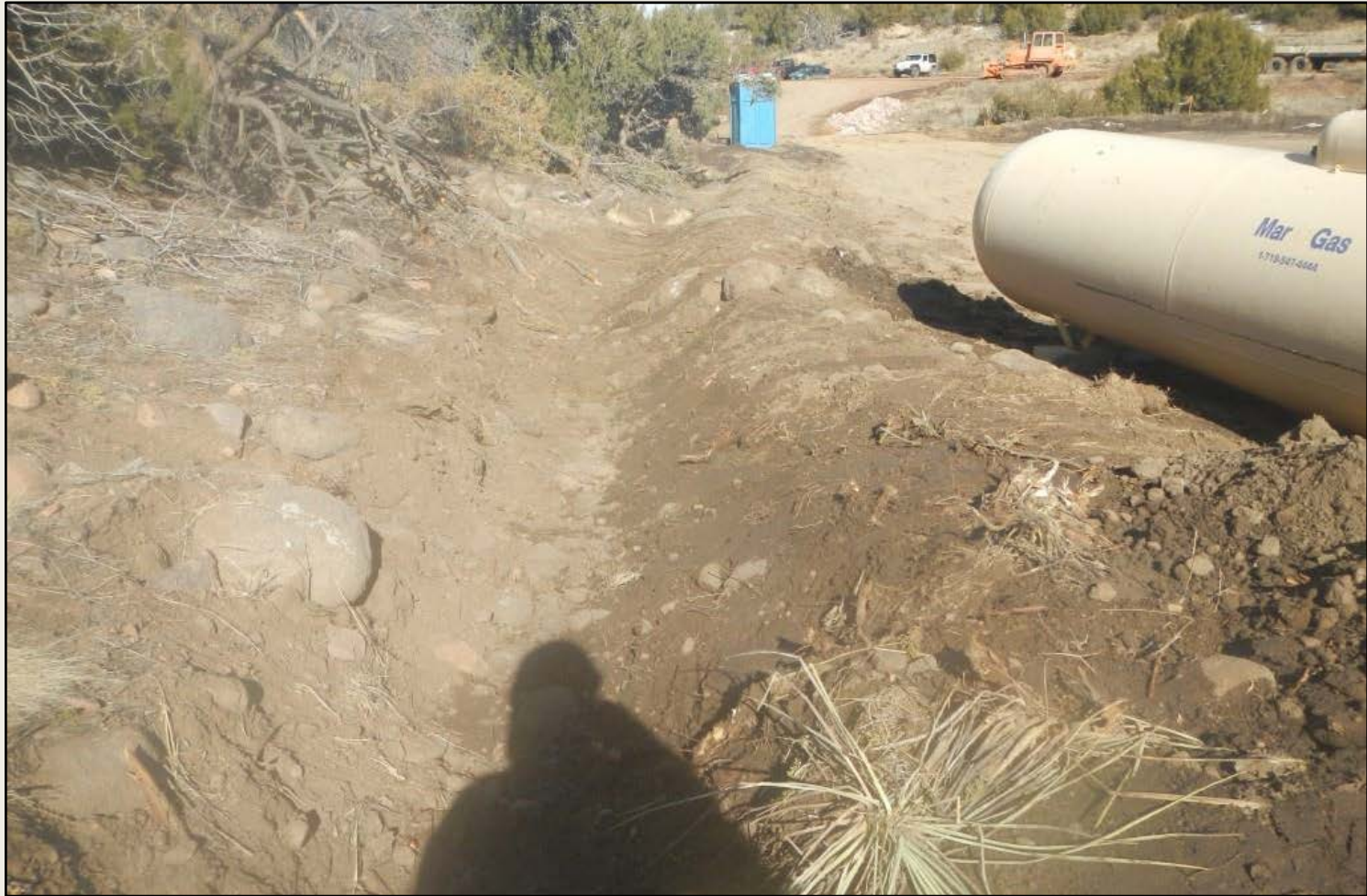
Photo 9. View of the northwestern project area from the northwestern corner facing eastward. As described above, diversion not properly stabilized or properly installed.
