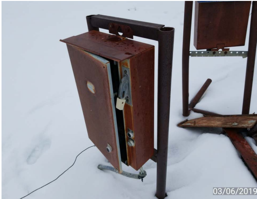
Photo 3. Electric panel not closed.
