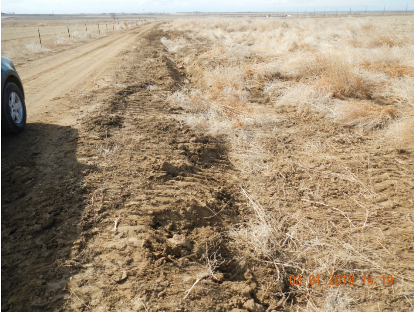
Photo 3. Photo taken from the access road, facing West. Photo depicts recent pipeline removal work on the north side of the road.
