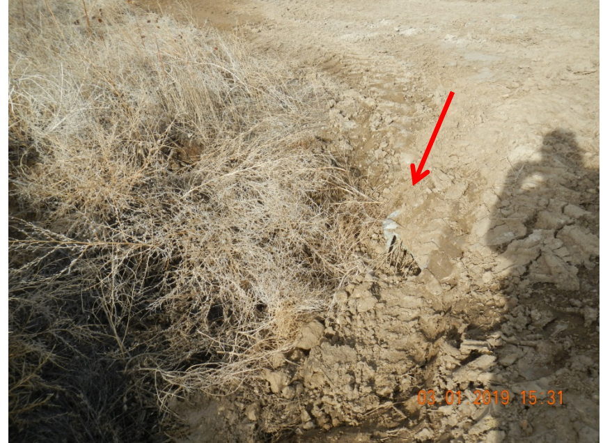
Photo 10. Photo taken from the western perimeter of the location. Photo depicts the culvert that was damaged/crushed during the pipeline removal work.
