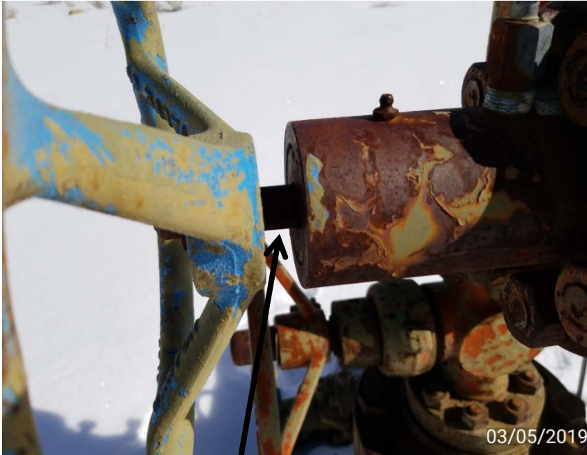
Photo 3. Gas leak #2.
