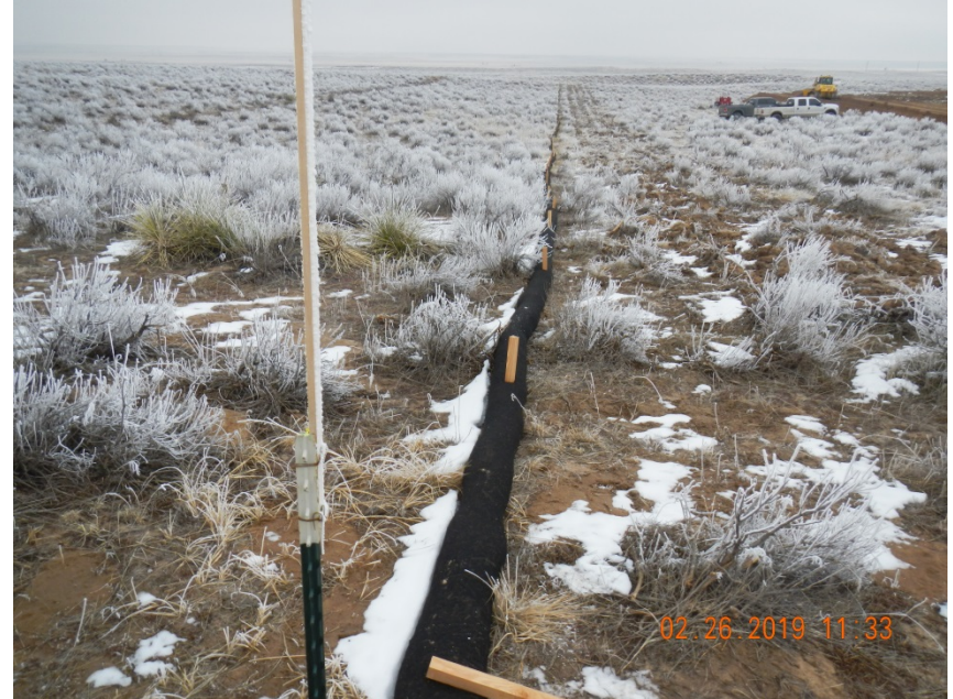
Photo 2. Photo taken from the northwestern perimeter of the location, facing North. Photo illustrates a filtrex BMP that has been installed around the perimeter of the location.
