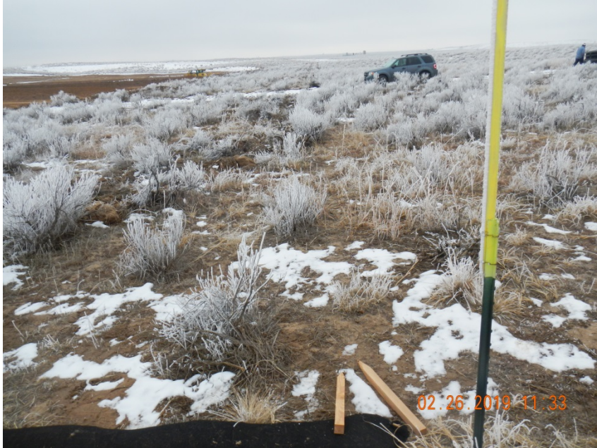
Photo 1. Photo taken from the northwestern perimeter of the location, facing South. Photo illustrates a filtrex BMP that has been installed around the perimeter of the location. However it appears the Operator has left a gap in the Filtrex along northwestern perimeter. BMPs are not in proper functioning condition at the time of this inspection.
