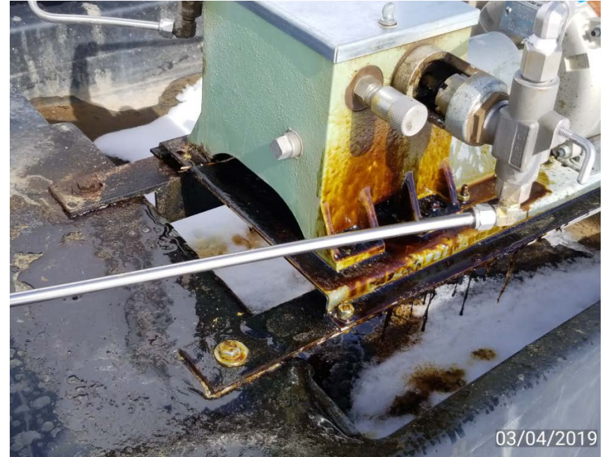
Photo 2. Inhibitor pump leaking fluid.
