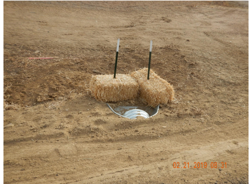
Photo 2. Photo taken along the access road, facing West. Photo illustrates straw bales used as stabilized outlets along the culverts.
