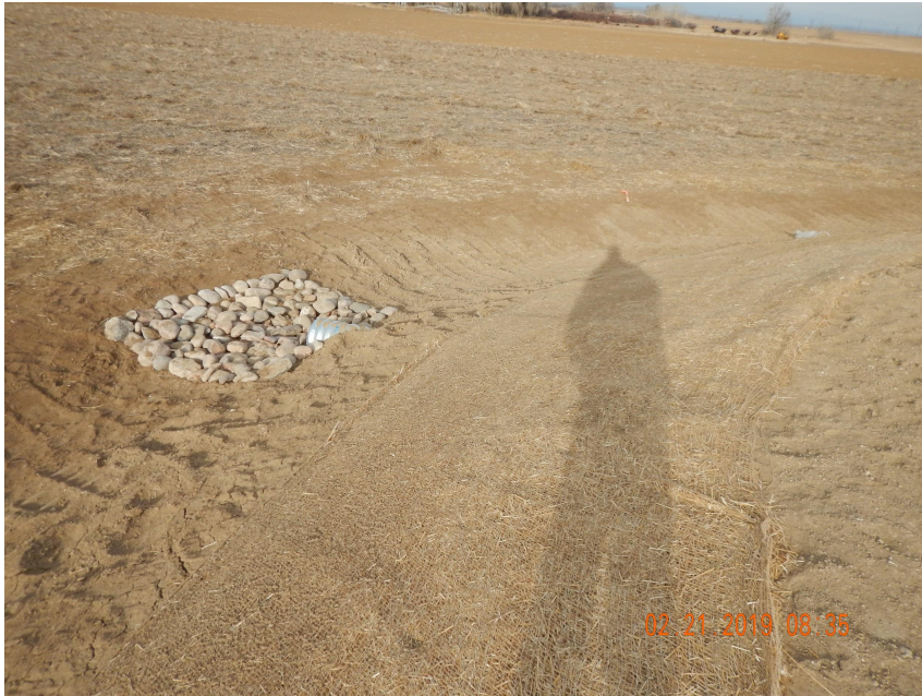
Photo 7. Photo taken from the southwestern perimeter of the location, facing West. Photo illustrates the stabilized outlet from the retention area. Erosion control blankets have been installed along portions of fill slopes.
