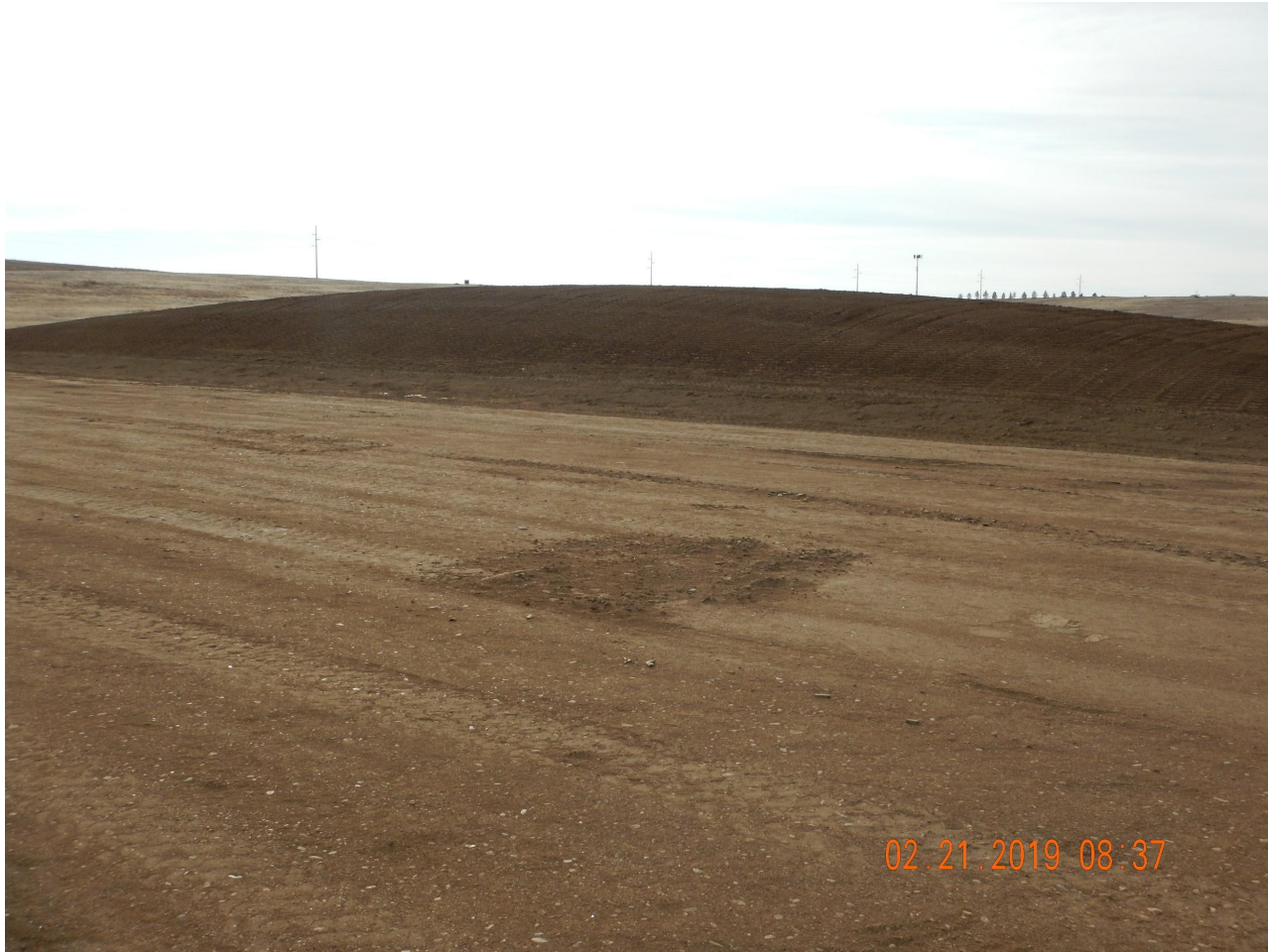
Photo 11. Photo taken from the southern well pad, facing South. Photo illustrates the topsoil stockpile which has been temporarily stabilized with equipment tracking.
