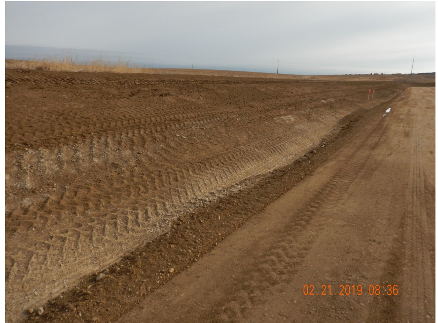
Photo 10. Photo taken from the northern perimeter of the well pad, facing East. Operator shall stabilize cut slopes.
