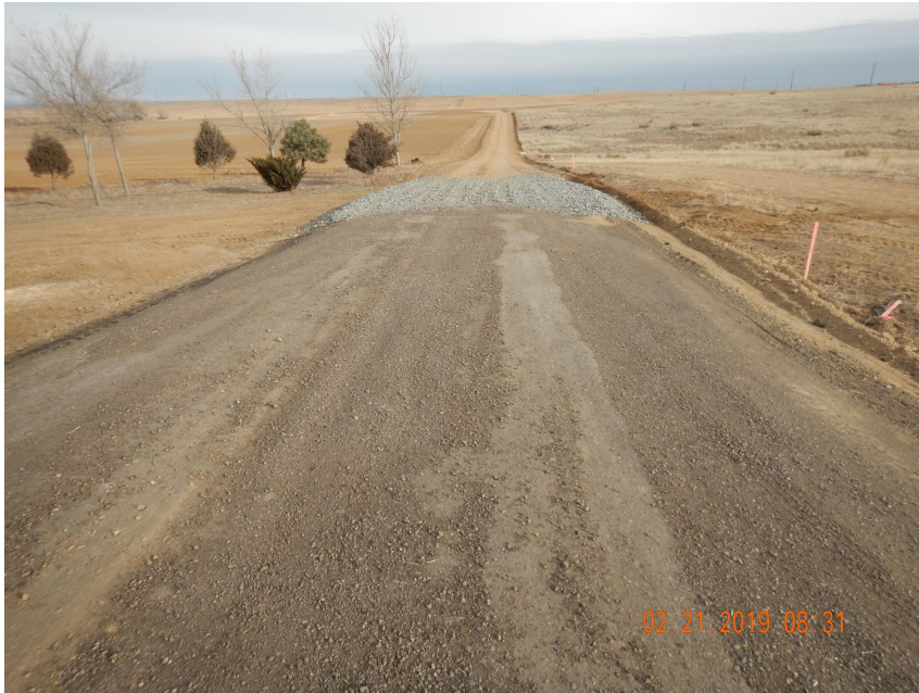
Photo 1. Photo taken from the entrance of the location off HWY 14, facing North. Photo illustrates vehicle track device BMPs have been installed and appear to be in proper functioning condition.
