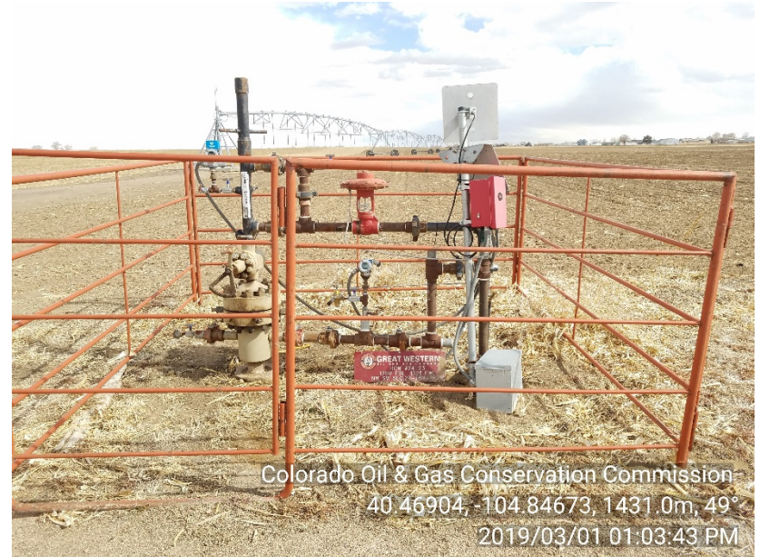
Photo #2 HCW 24-23 (05-123-31497) Wellsite Shut-In | SI Emergency number NOT posted Sign not attached
