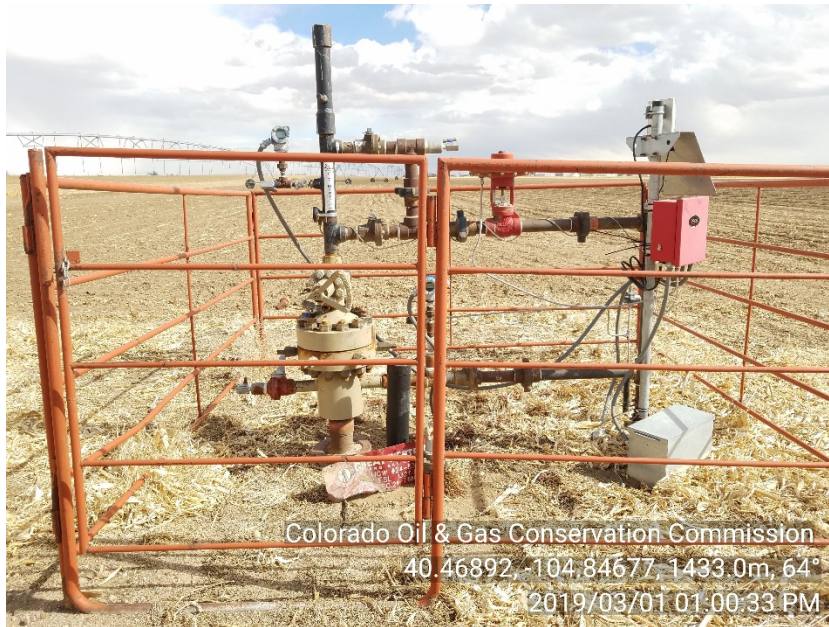
Photo #3 HCW 24-53 (05-123-31501) Wellsite Shut-In | SI Emergency number NOT posted Sign not attached, bent
