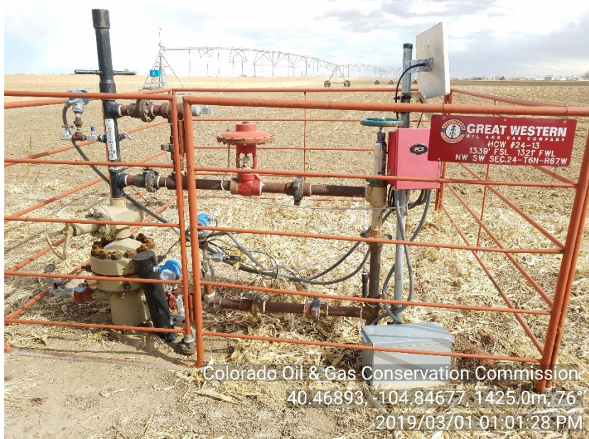
Photo #1 HCW 24-13 (05-123-31500) Wellsite Shut-In | SI Emergency number NOT posted
