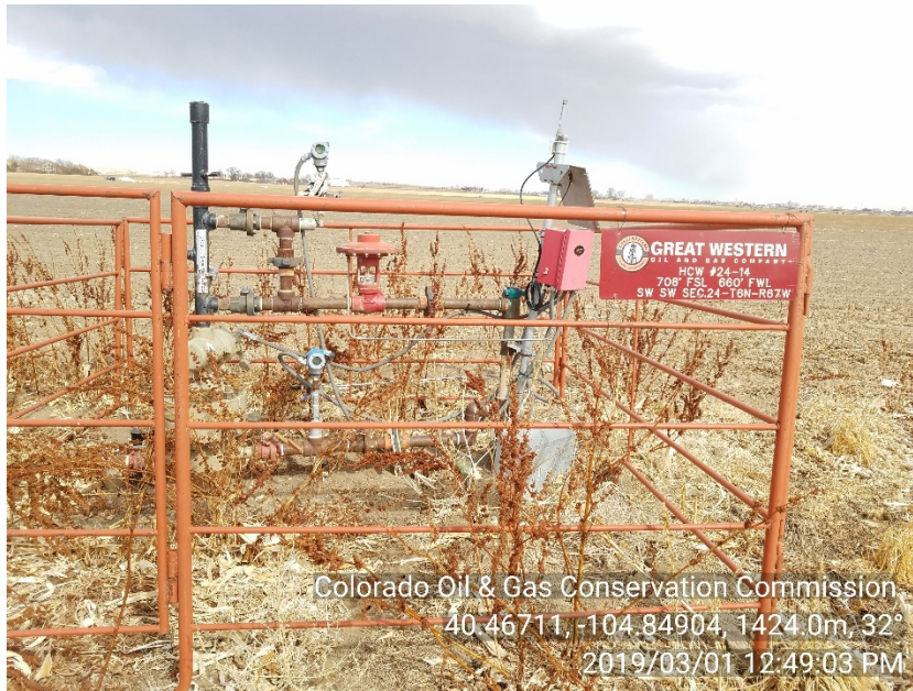
Photo #3 HCW 24-14 (05-123-31498) Wellsite Shut-In | SI Emergency number NOT posted Weeds
