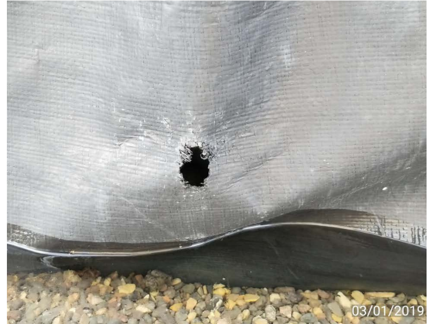
Photo 2. Hole in liner.
