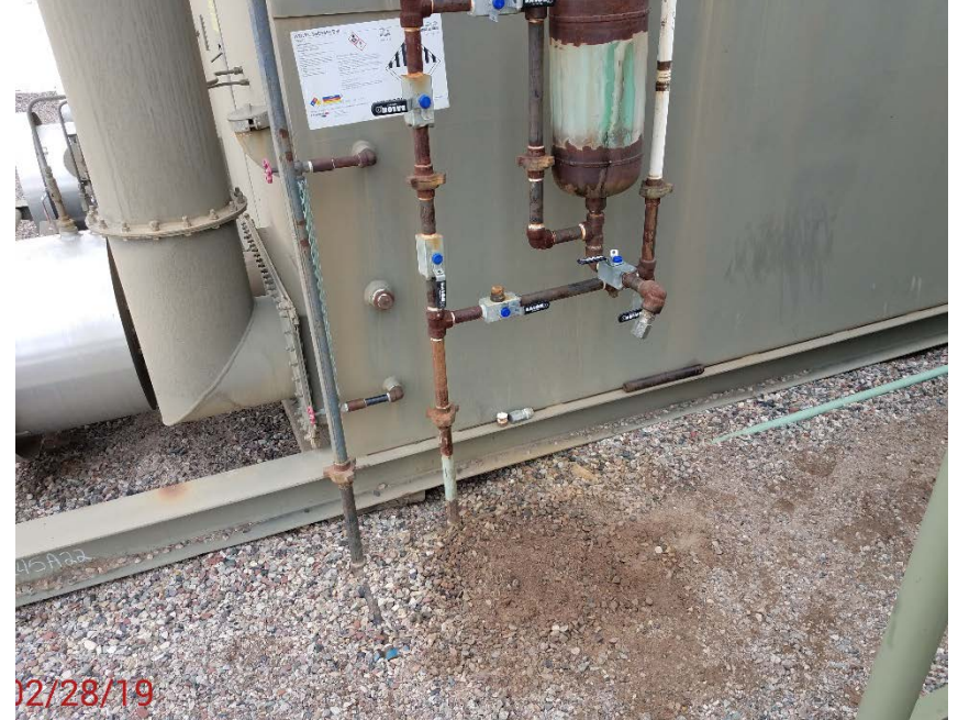
Location Photo #4, Stained ground underneath the scrubber pot.
