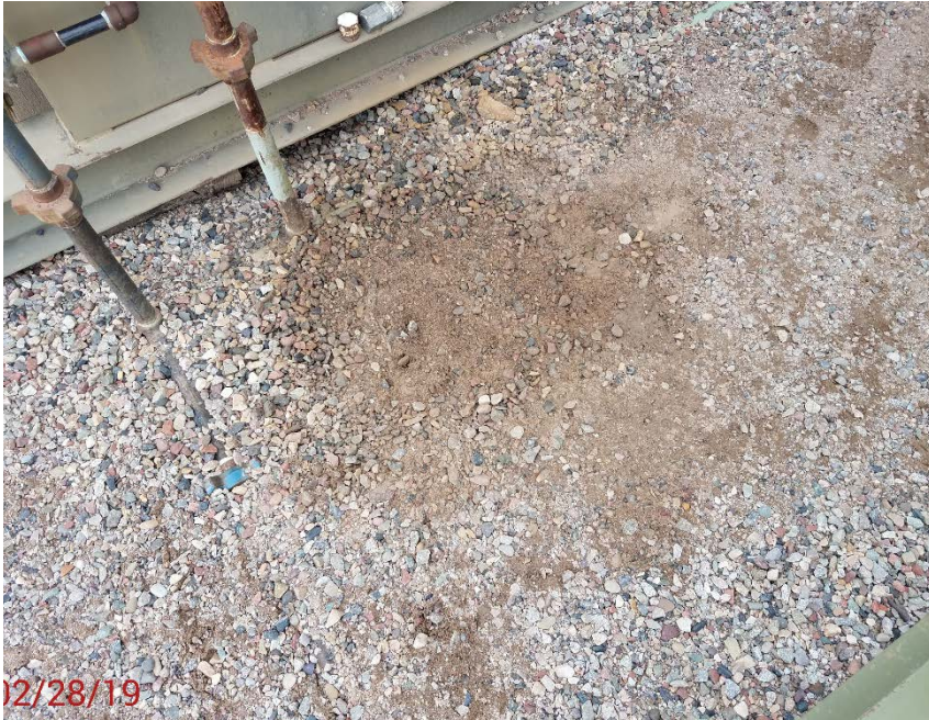
Location Photo #5, stained ground underneath scrubberpot.
