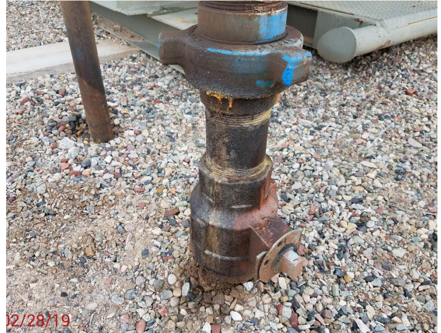
Location Photo #6, leaking fitting on unit 23D
