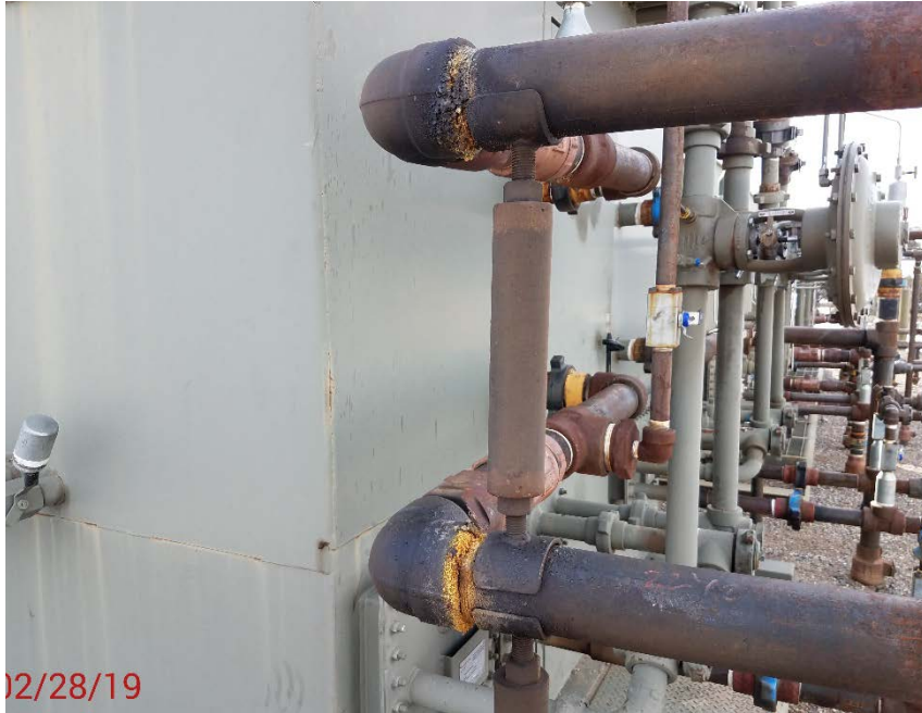
Location Photo #5, 2 leaking fittings on unit 23D
