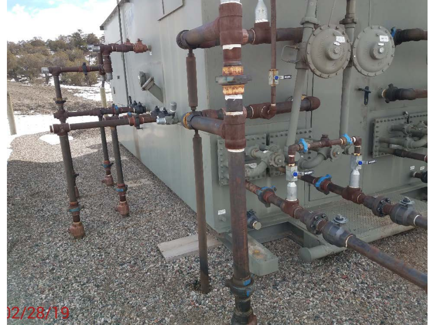
Location Photo #4, Leaking fittings on unit 23D
