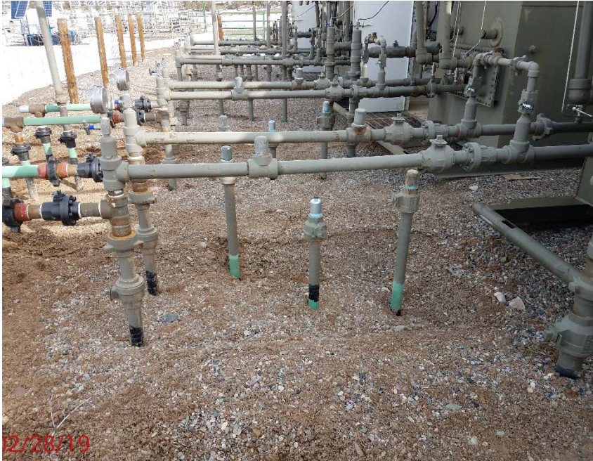
Location Photo #5, 6 unmarked/unused flow line risers.
