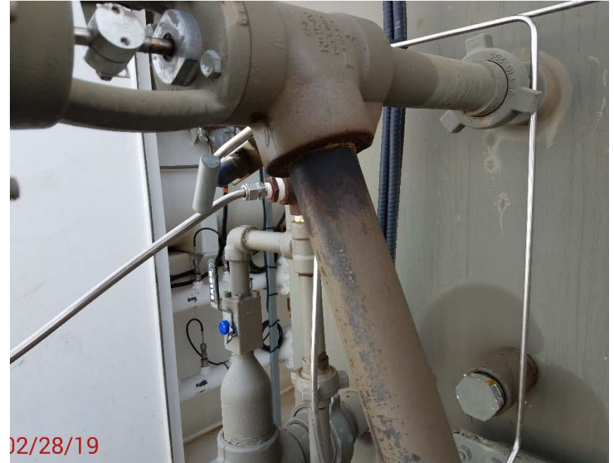
Location Photo #8, leaking fittings below the kimray on unit 44D
