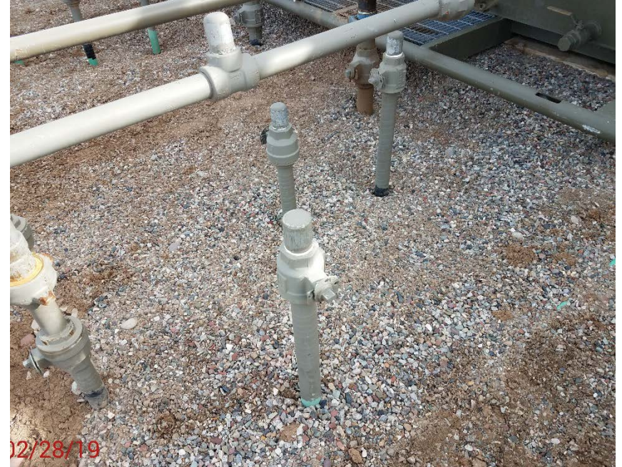
Location Photo #4, 3 unmarked/unused flow line risers.
