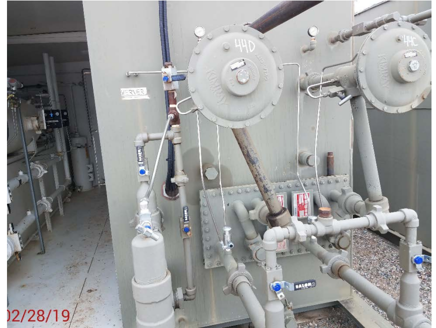
Location Photo #6 unit 44D has leaking fittings.
