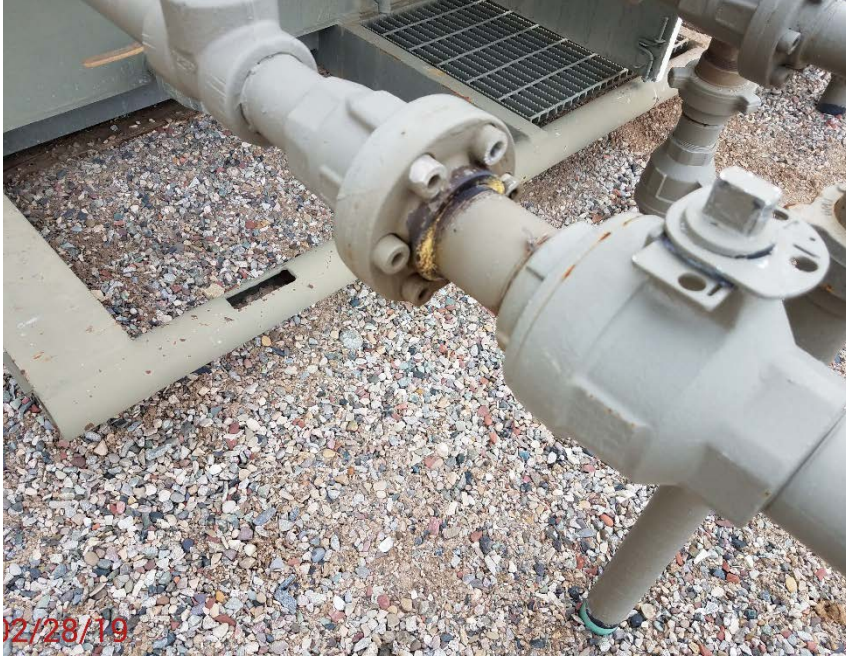
Location Photo #11, leaking fitting at check valve on unit 44B
