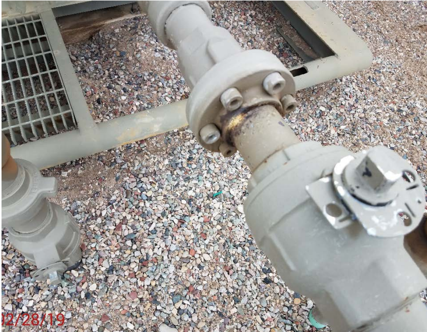
Location Photo #9, leaking fitting at the check valve unit 44D
