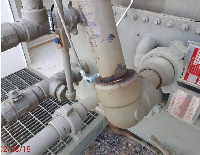
Location Photo #7, leaking fittings below the kimray on unit 44D
