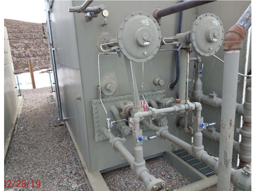
Location Photo #10, Leaking fitting on unit 44B.
