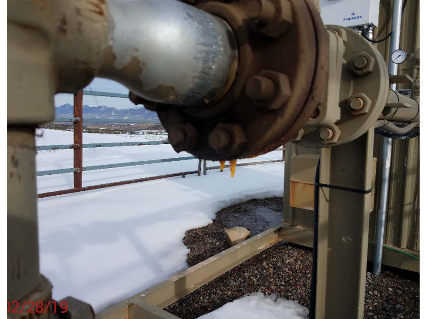
Location Photo #4, Leaking flange on inlet line to meter run
