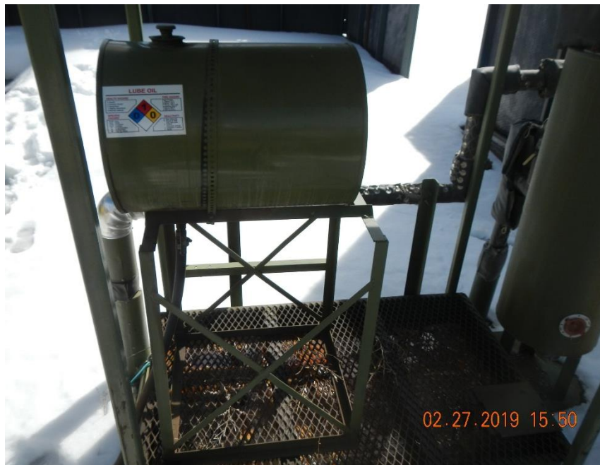
Lube oil container on secondary containment. Secondary containment is almost full.
