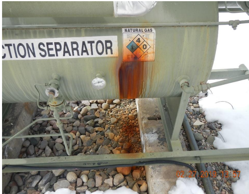
Rust colored staining present on vessel and gravel beneath aluminum elbow.
