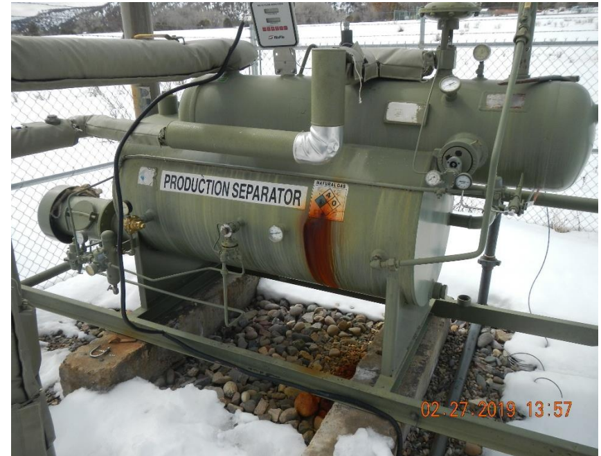
Horizontal heated separator has rust colored staining below aluminum elbow.
