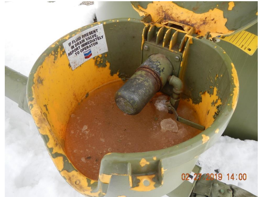
Drip pot on AST load out line with ice and fluids present.
