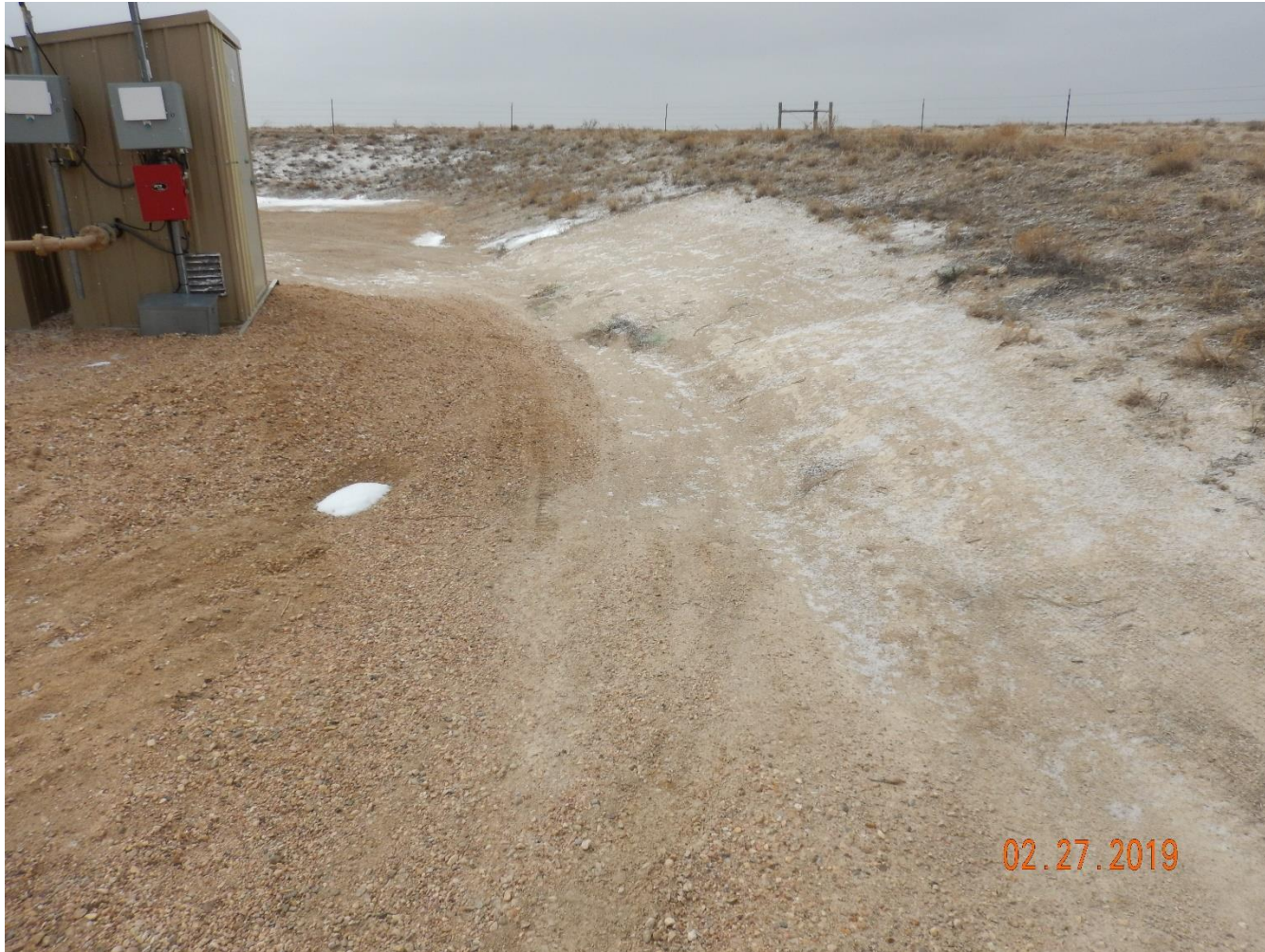
Photo 11: Photo taken from the west end of the location. Photo shows areas where operator appears to have traveled from the location onto slopes of the interim areas.
