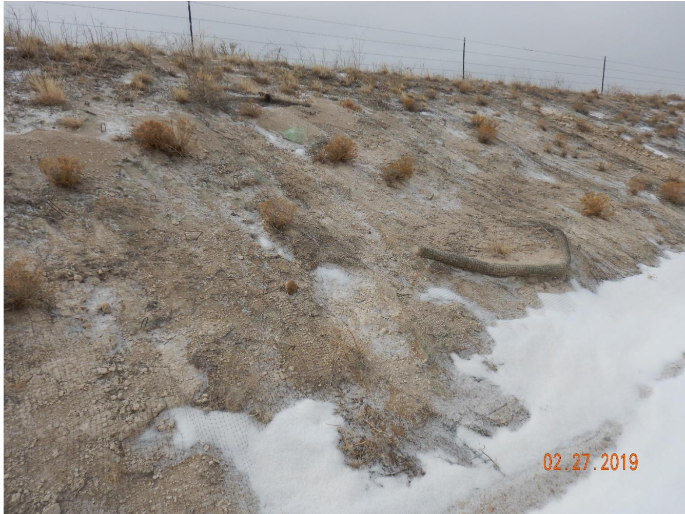
Photo 13: Photo taken from the slopes of the interim areas on the south end of the location, facing southwest. Photo shows slopes remains predominantly bare and exposed soil with little desirable perennial vegetative establishment. Photo also shows the erosion blankets/netting along slopes are in disrepair and no longer in proper functioning condition.
