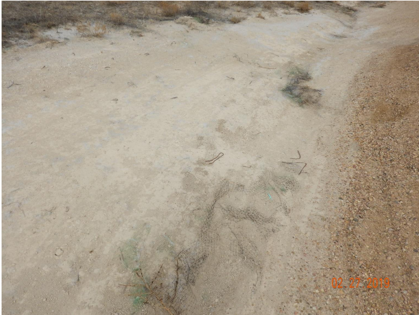
Photo 12: Photo taken from the slopes of the interim areas on the southwest end of the location. Photo shows slopes remains predominantly bare and exposed soil with little desirable perennial vegetative establishment. Photo also shows the erosion blankets/netting along slopes are in disrepair and no longer in proper functioning condition.
