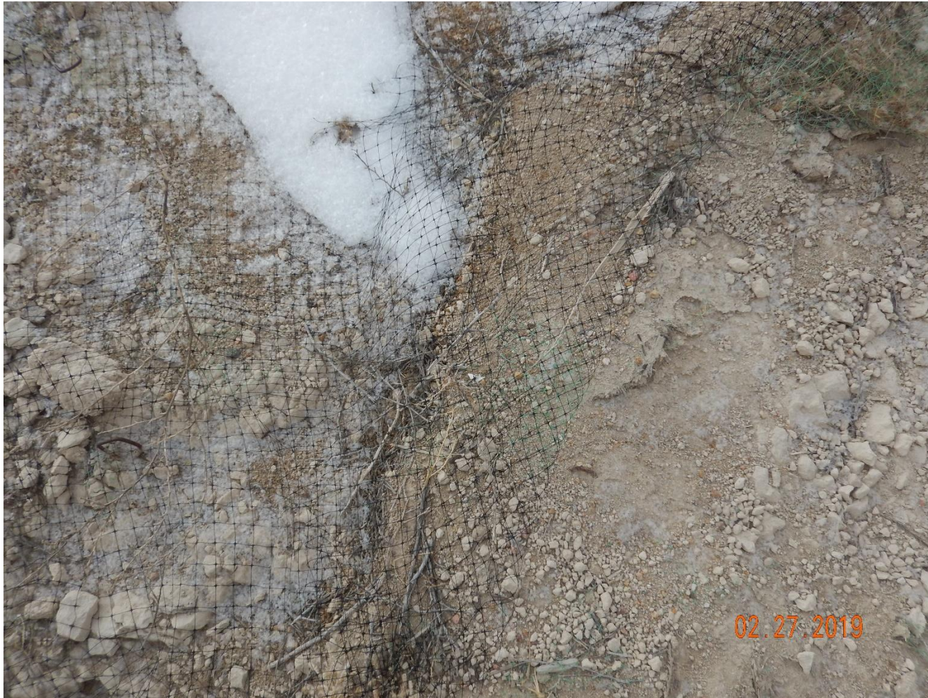
Photo 14: Photo taken from the slopes of the interim areas on the southwest end of the location. Photo shows the erosion blankets/netting along slopes are in disrepair and no longer in proper functioning condition.
