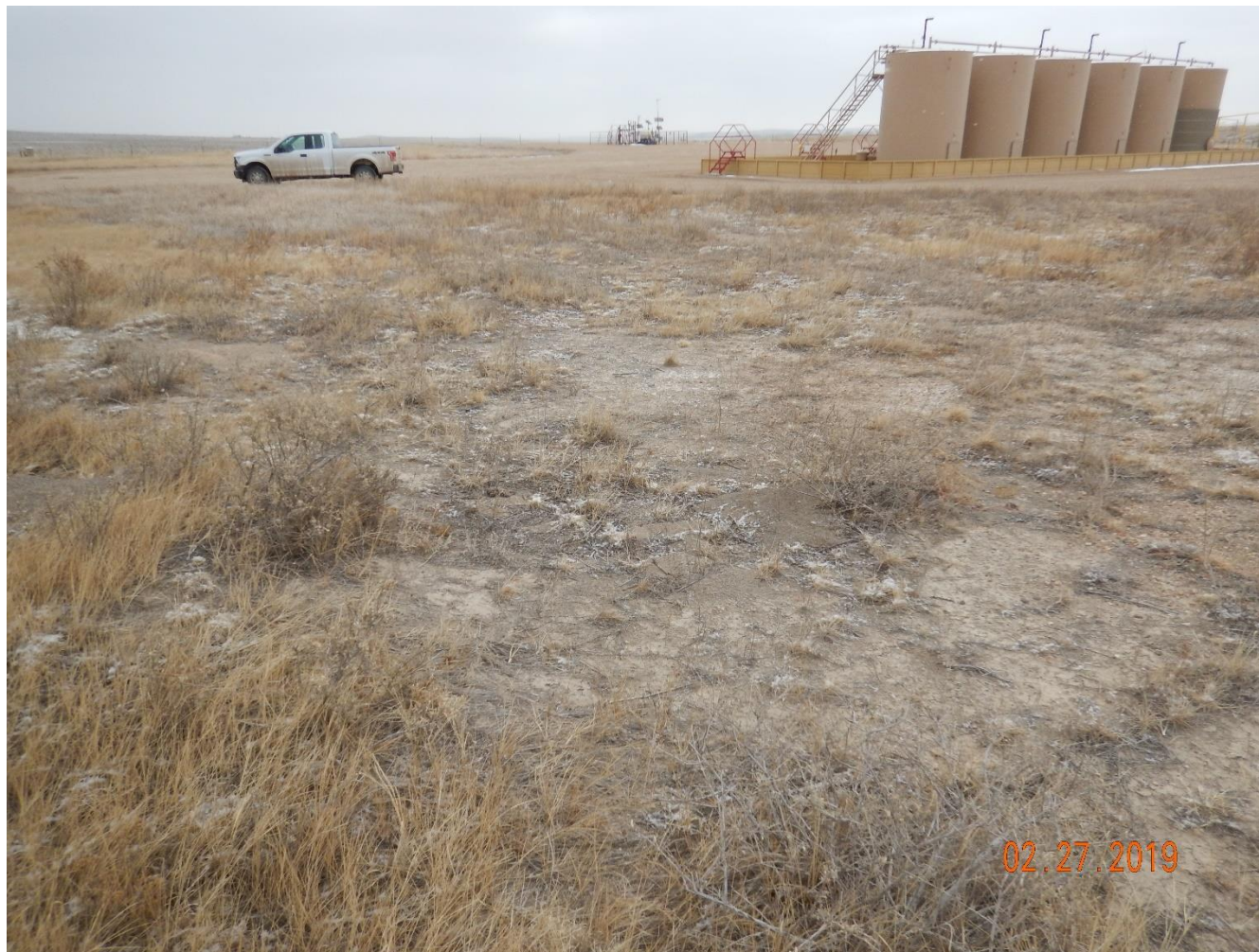
Photo 7: Photo taken from the northwest end of the location, facing southeast. Photo shows interim areas of the location are predominantly bare and exposed soil, or undesirable weedy plant species such as Kochia and Salsola sp. Areas are not progressing towards reclamation requirements.
