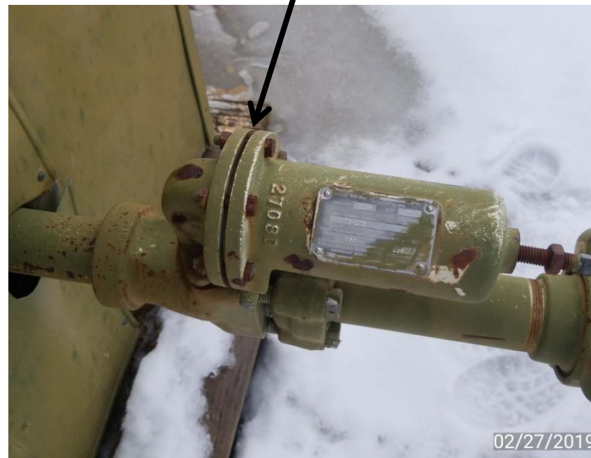
Photo 2. Gas leak at flange next to gas meter building.
