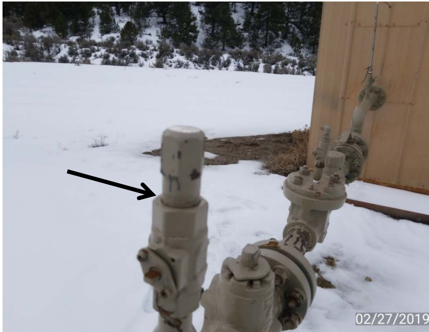
Photo 7. Gas leak through threads of bull plug on gas meter line.
